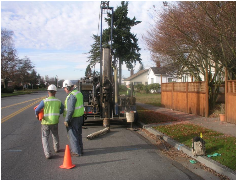
Plate 2. Looking west along 3 rd Street near 47 th Avenue NE. The drill rig is set up to drill boring B-8.
