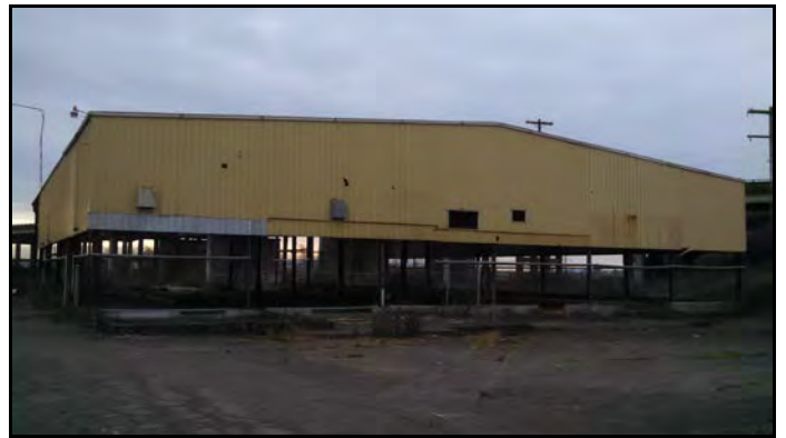
View of the vacant small log sawmill building, facing south.
