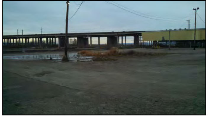
View of the central portion of the Subject Property, facing southwest.
