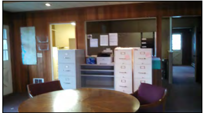
Typical interior view of the office building on the northeast portion of the Subject Property.
