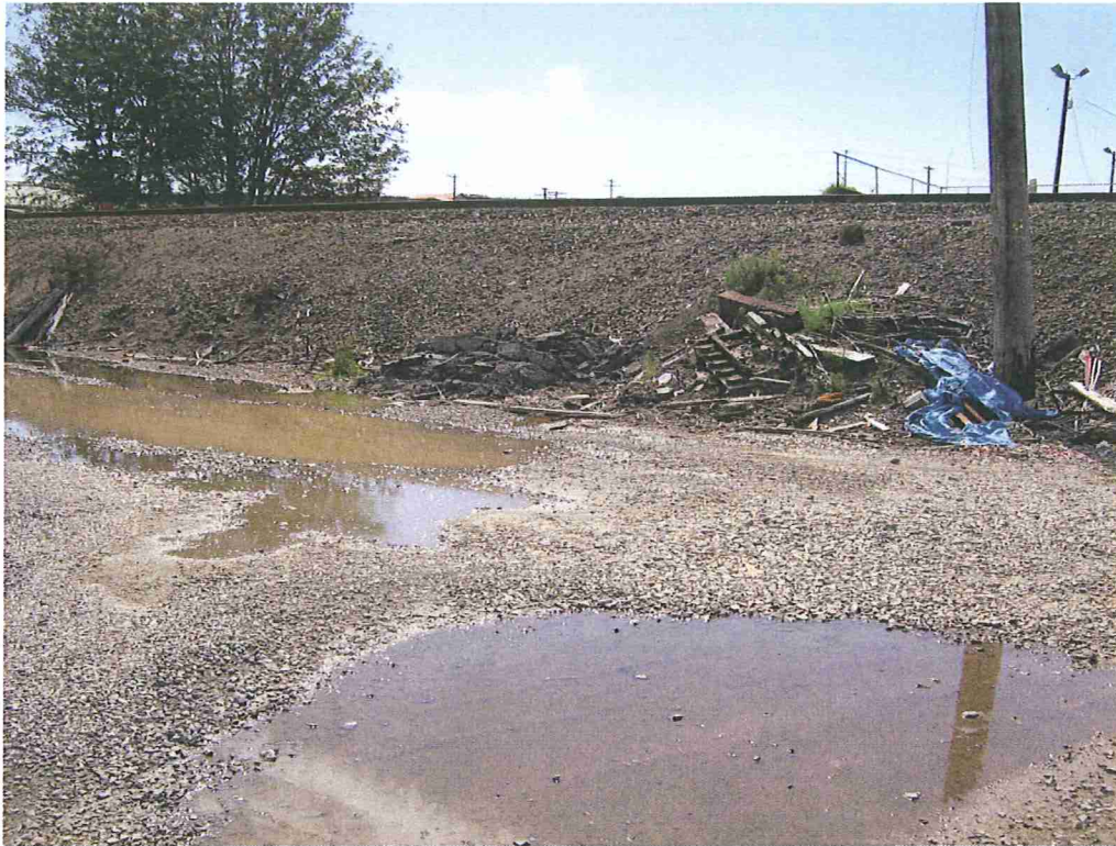
Photograph of debris piles observed on along the western boundary of the subject property. Viewing to the west.
