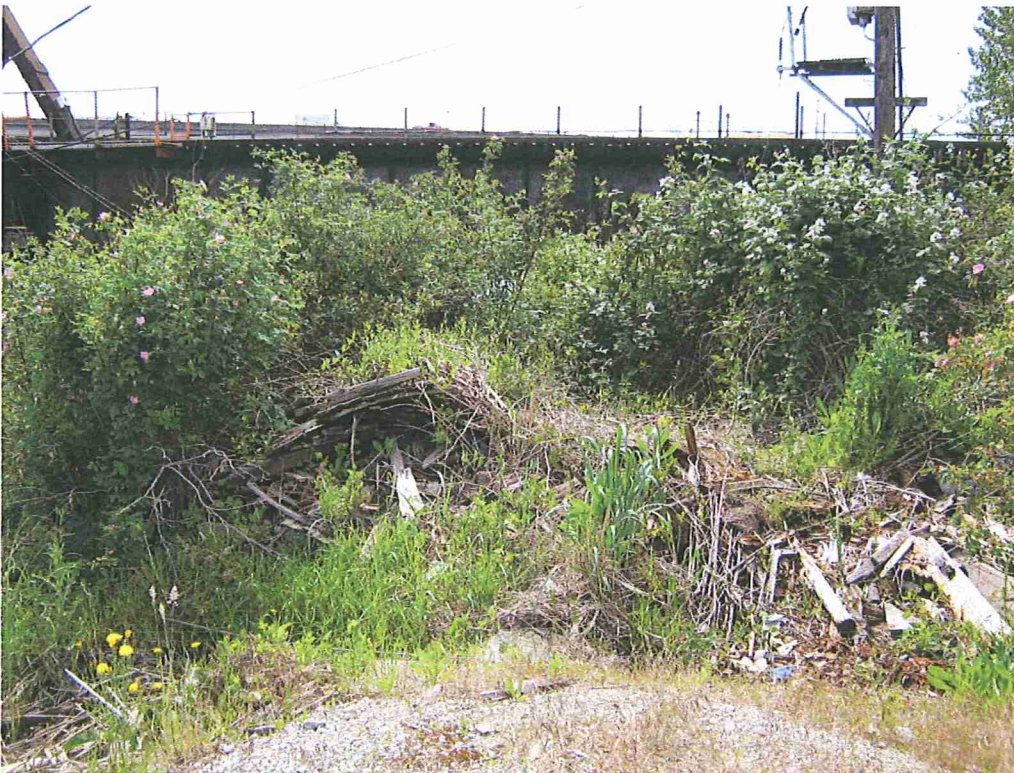
Photograph of a building materials debris pile located on the northwestern portion of the subject property. Viewing to the southwest.
