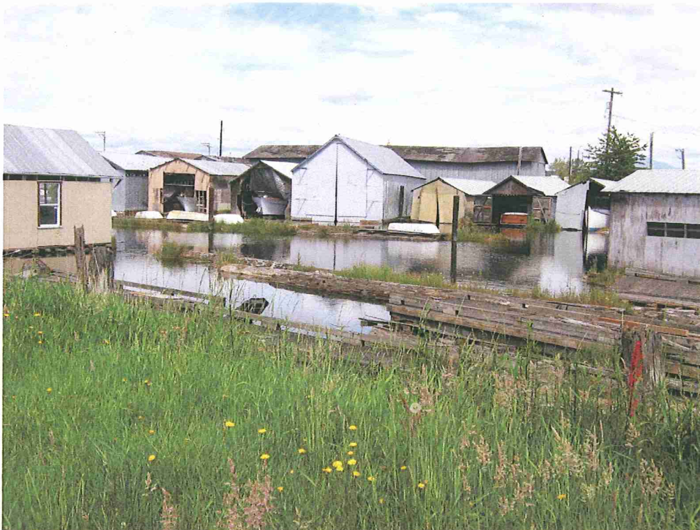
Photograph of the boat houses located on the eastern portion of the subject property. Viewing to the northeast.
