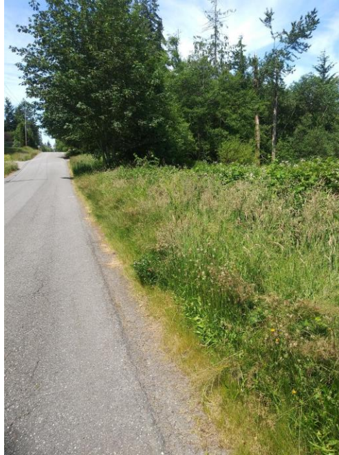
Image 1: Low point along 60 th St NE. Site runoff drains to this point and flows north and east.
