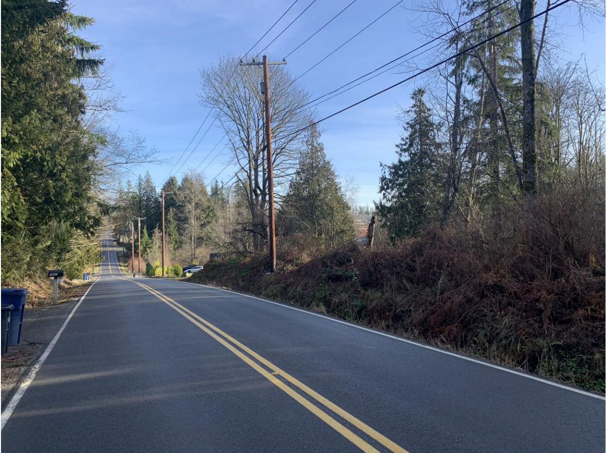
Image 1: Facing easterly near the NW corner of the project site where road and topography slopes east towards the low point at the King Creek inlet to the site. Negligible upstream runoff north of 44 th St NE. See Image 6 for description of upstream runoff from the west.
