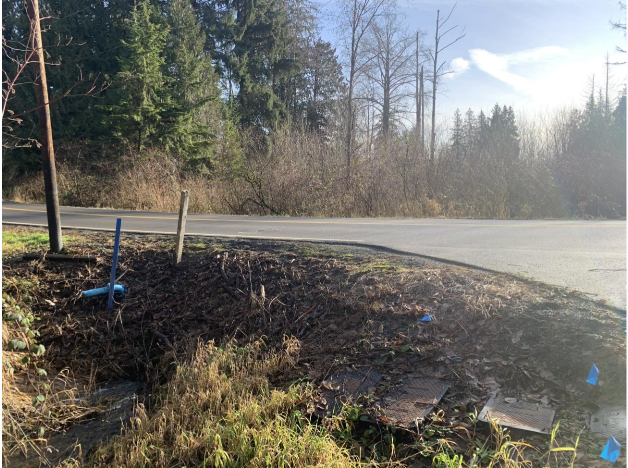
Image 2: Facing southerly at the King Creek inlet to the project site at a low point along 44 th St NE near the NE corner of project site. King Creek continues through the project site wetland areas near the eastern edge before discharging from the site at the southern edge.
