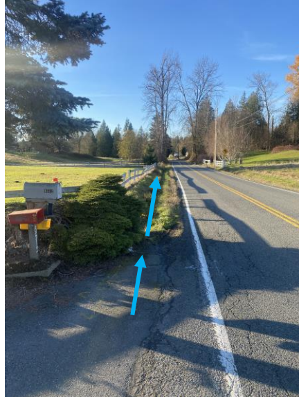
Image 2: Facing west along E Sunnyside School Rd where Flowpath 1 continues in a roadside ditch
