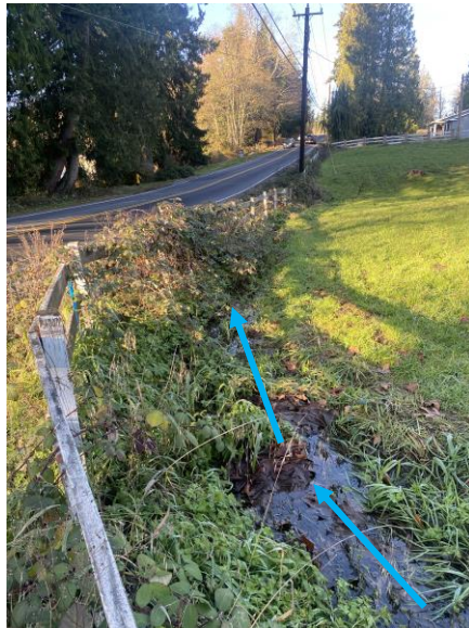
Image 8: Intersection of E Sunnyside School Rd and 83 rd Ave NE
