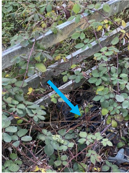
Image 9: Intersection of E Sunnyside School Rd and 83 rd Ave NE where flow crosses west under 83 rd via culvert
