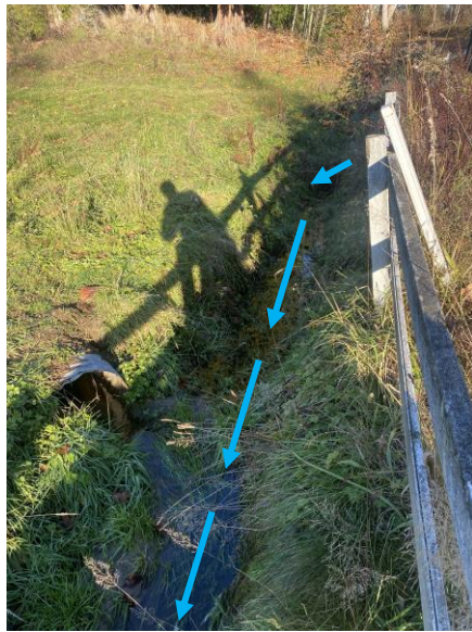
Image 6: north side of E Sunnyside School Rd where channelized flow continues west
