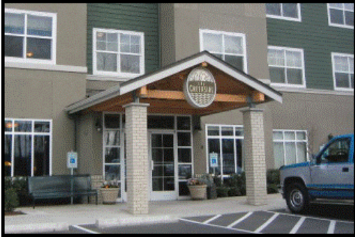
Figure 18 – A distinct, weather-protected primary building entrance.
