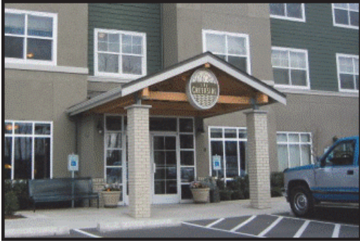
Figure 18 – A distinct, weather-protected primary building entrance.
