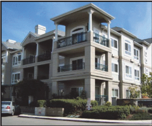
Figure 15 – A residential courtyard providing semi-private patio spaces adjacent to individual units.
