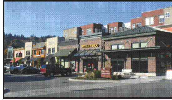
Figure 9 – This development uses a variety of roof forms and heights, different weather protection features, changing building materials and colors, and a modest amount of horizontal building modulation to reduce the overall architectural scale into smaller “storefront” components.
