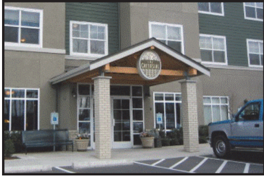
Figure 18 – A distinct, weather-protected primary building entrance.
