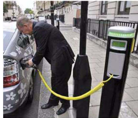
On-street charging near end of block.
