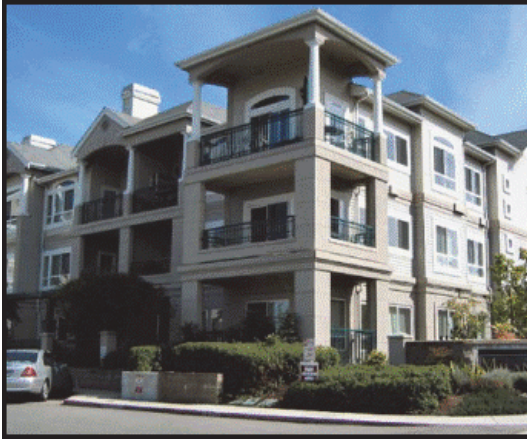
Figure 21 – A residential courtyard providing semi-private patio spaces adjacent to individual units.
