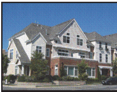
Figure 4 – An example of articulating a building’s top, middle, and bottom by utilizing brick on the ground floor, defined window patterns and articulation treatments on upper floors, and a distinctive roofline.
