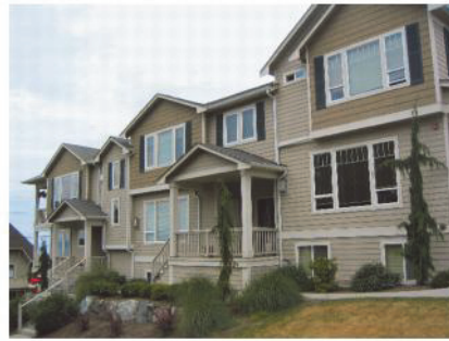
Figure 7 – Weather protection that articulates the front facade is provided.
