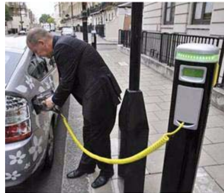
On-street charging near end of block.
