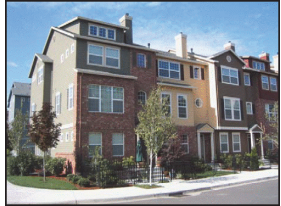
Figure 10 – This building uses brick for more than 10 percent of the facade, a decorative mix of materials and colors, decorative entries, and decorative windows to add visual interest.
