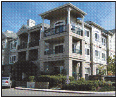
Figure 2 – An example of balconies that have been integrated into the architecture of the building.
