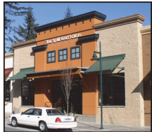
Figure 15 – This storefront effectively combines EIFS and concrete block with wood trim and metal detailing.
