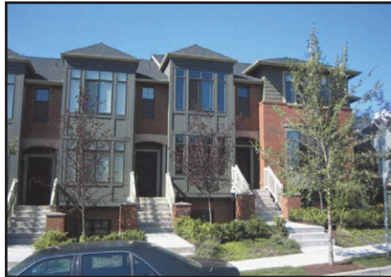
Figure 8 – Ground floor residential units directly accessible to the street with landscaping defining the entry.
