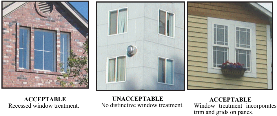
Figure 11 – Acceptable and unacceptable window treatments.
