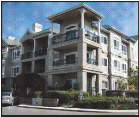
Figure 2 – An example of balconies that have been integrated into the architecture of the building.
