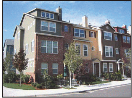
Figure 10 – This building uses brick for more than 10 percent of the facade, a decorative mix of materials and colors, decorative entries, and decorative windows to add visual interest.
