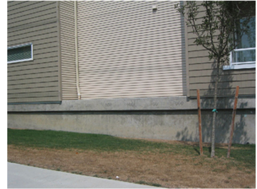
Figure 8-3. Exposed foundations like this should be landscaped with shrubs and other plantings for screening
