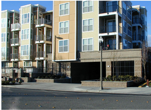
Figure 5-2. A good example of a parking garage entrance for a mixed-use development.
