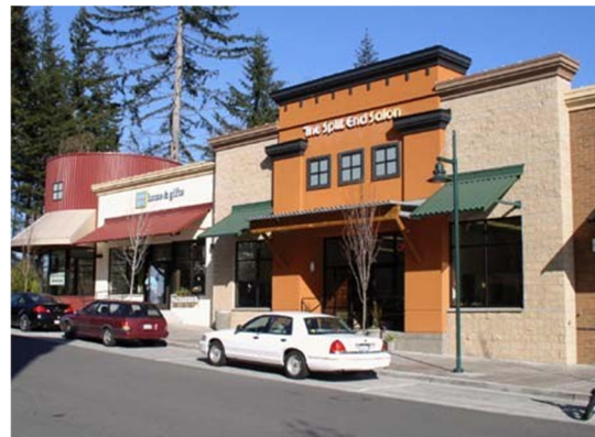
Figure 7-9. This building utilizes a number of methods to reduce its perceived bulk.
