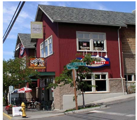
Figure 7-25. This building features metal siding with visible corner trim and concrete block closer to the ground level.
