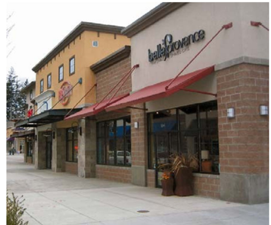
Figure 7-24. An example of concrete block effectively used with EIFS and metal awnings.
