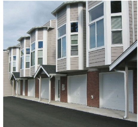
Figure 7-3. A bad townhouse example with no landscaping adjacent to the entry.
