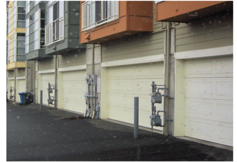
Figure 8-6. Exposed utility meters like this will not be allowed.
