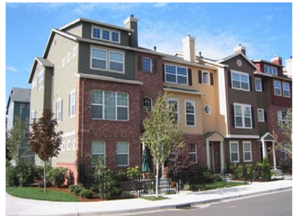
Figure 7-20. This building uses brick for more than 10% of the façade, a decorative mix of materials and colors, decorative entries, and decorative windows to add visual interest.
