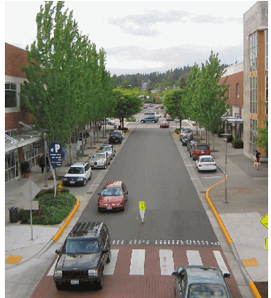
Figure 5-1. Internal access road designed to look and function like a public street. Note on-street parking, lighting, street trees, and sidewalks.
