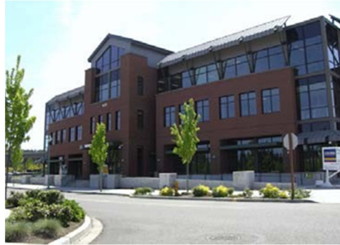
Figure 7-16. The prominent vertical element of this building effectively breaks up the perceived scale of the building and adds visual interest.
