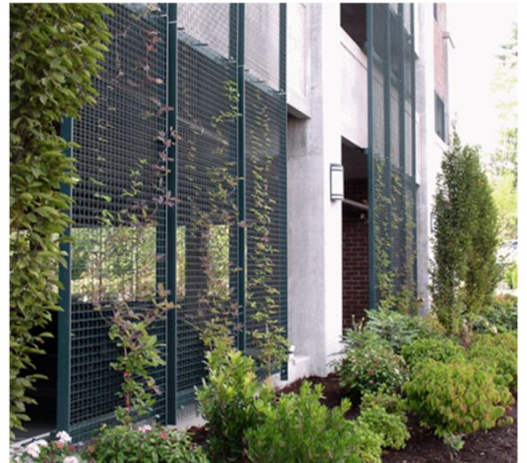
Figure 5-3. A good parking garage example with landscaping elements to screen cars and provide visual interest
