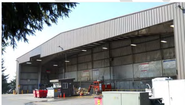
North County Recycling and Transfer Station
