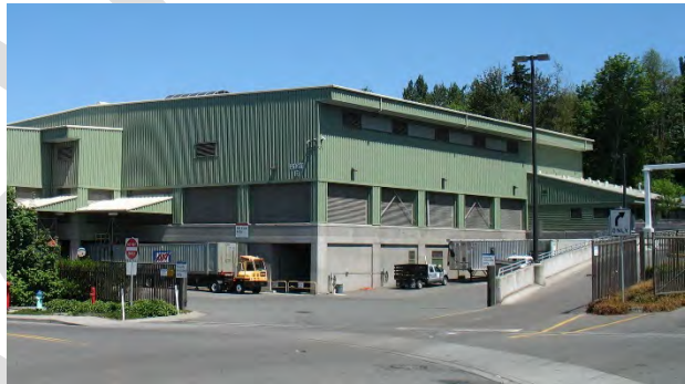
Southwest Recycling and Transfer Station
