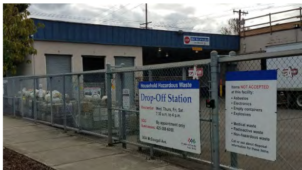
Moderate Risk Waste Facility
