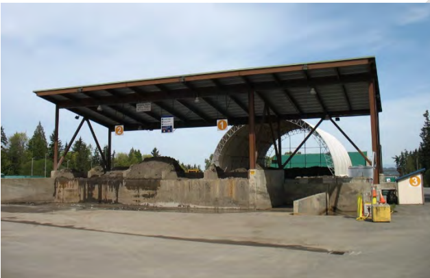
Vactor Decant Waste Facility at Cathcart
