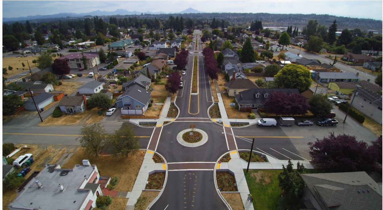
Above image of Third Street improvements and LID
