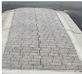
STAMPED MODULAR STONE CONCRETE IN MEDIAN ISLANDS
