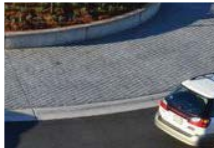
STAMPED MODULAR STONE CONCRETE IN ROUNDABOUT APRON
