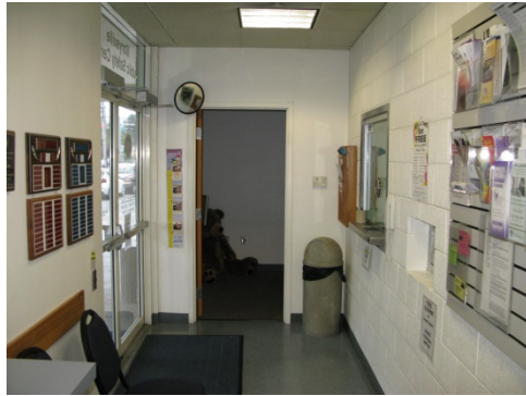
Inadequate Public Lobby
