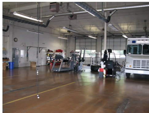
Fire Equipment Bay
