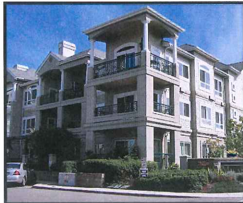
Figure 2– An example of balconies that have been integrated into the architecture of the building.
