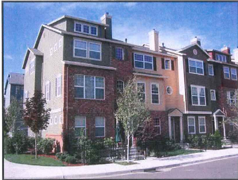
Figure 10 – This building uses brick for more than 10% of the facade, a decorative mix of materials and colors, decorative entries, and decorative windows to add visual interest.
