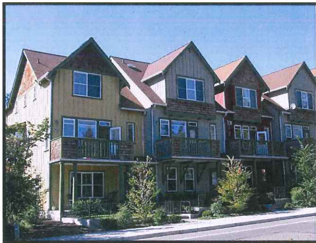
Figure 17 - Common open space for a townhouse development.
