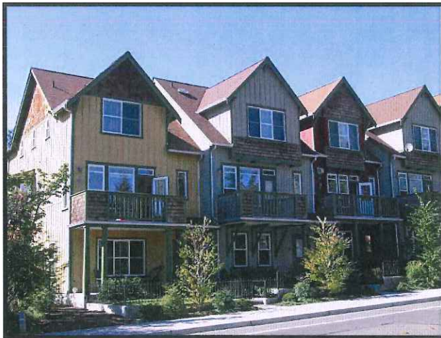
Figure 23 - Common open space for a townhouse development.
