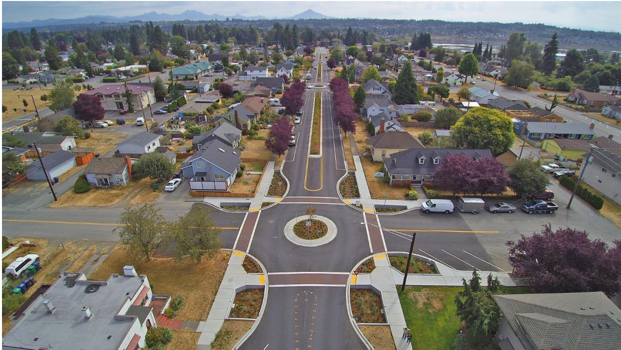
Figure 8. 3 rd St and Alder Ave in the downtown neighborhood.
