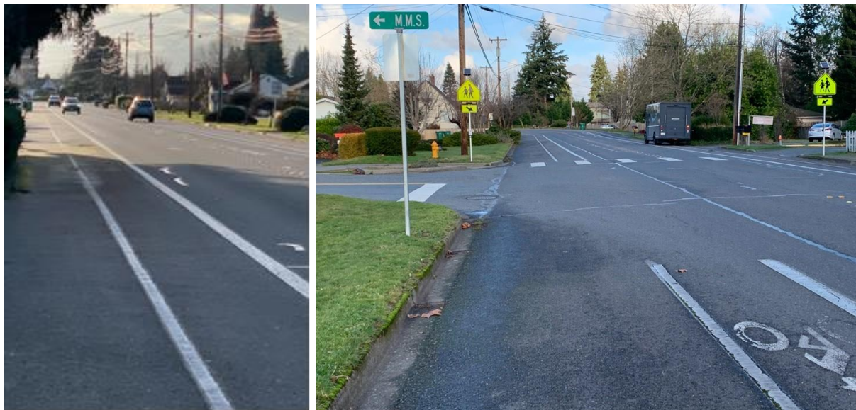
Figure 40. L-R: existing cross section; school crossing at 67 th St NE
