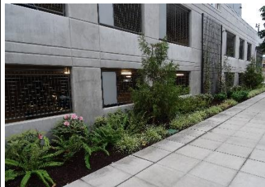
Parking garage with window openings
