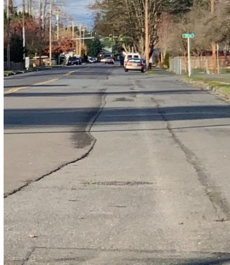
Figure 32. Quinn Ave north of 4th St
