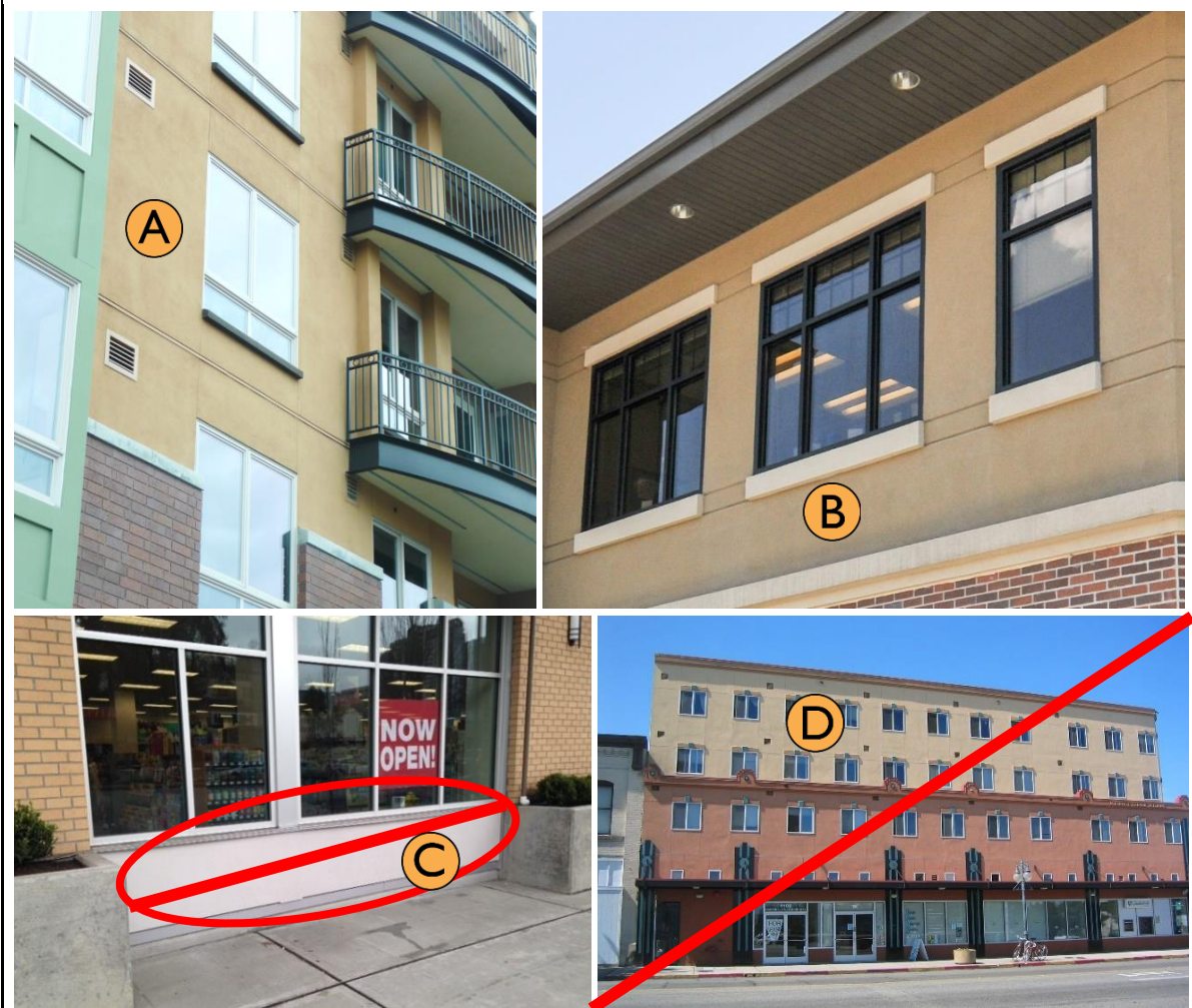
Figure 22C.080.530(c) Acceptable and unacceptable EIFS examples.
