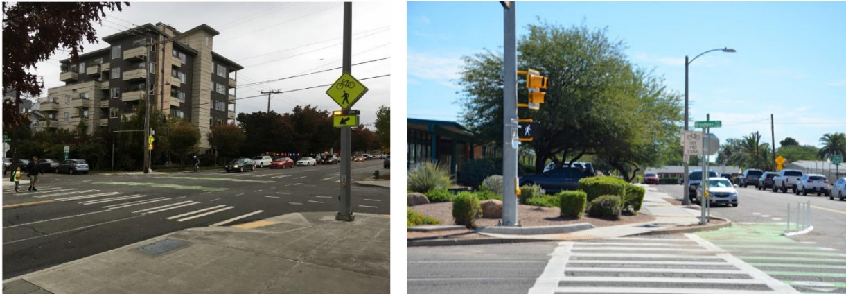
Figure 39. L-R: a rectangular rapid flashing beacon (RRFB); a high-intensity activated crosswalk (HAWK) beacon with bicycle accommodations.
