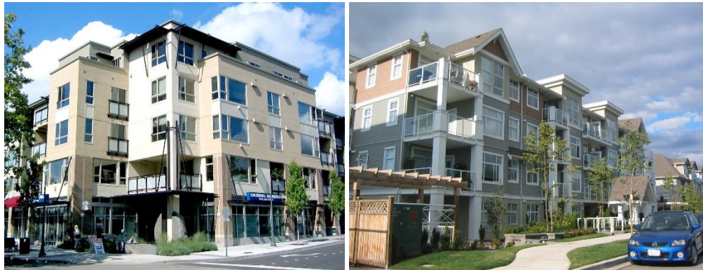
Figure 14.L-R: “four over one” mid-rise apartment building with ground floor shop; four-story apartment building
