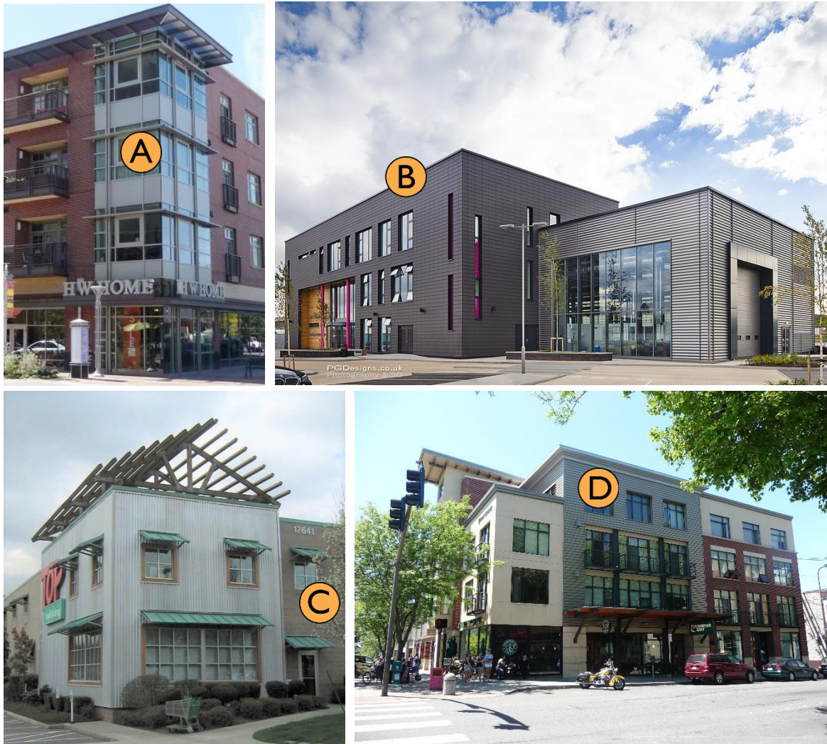
Figure 22C.080.530(2)(b) Acceptable metal siding examples
