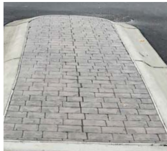
STAMPED MODULAR STONE CONCRETE IN MEDIAN ISLANDS
