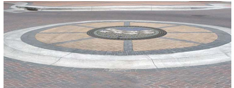
MOUNTABLE VEHICLE GRADE PAVERS (APPROX. 6"X6" CREAM/GRAY COLOR TONES) SET IN GEOMETRIC PATTERN WITH CENTER ART MEDALLION
