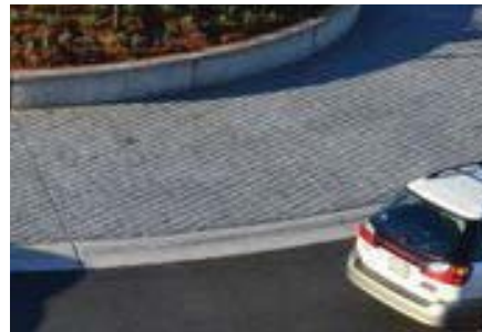
STAMPED MODULAR STONE CONCRETE IN ROUNDABOUT APRON
