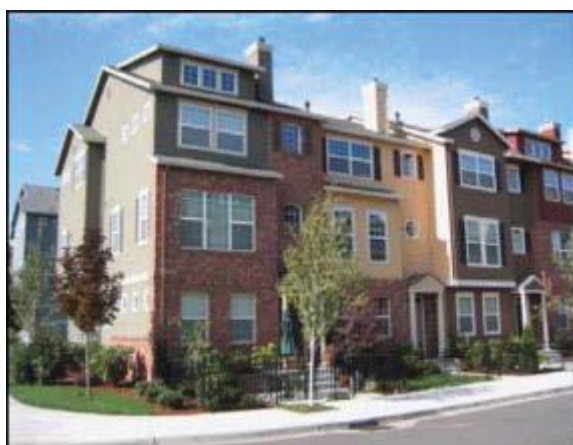
Figure 13 – This building uses brick for more than 10 percent of the facade, a decorative mix of materials and colors, decorative entries, and decorative windows to add visual interest.
