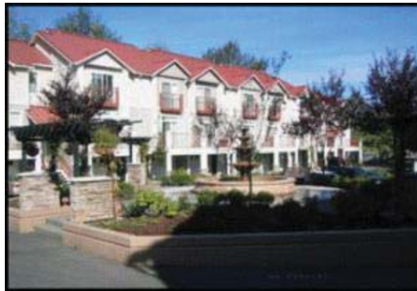
Figure C27 – These townhouses provide balconies and semi-private yard space
