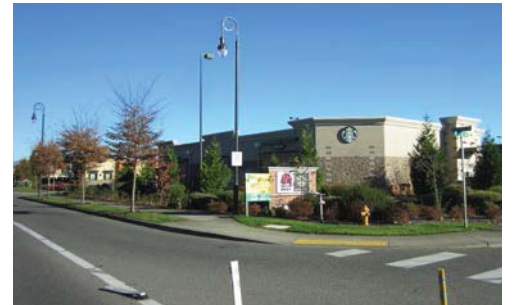
Figure 4. The Lakewood Crossing shopping area has quality landscaping and building design, but the development is scaled and oriented to the automobile, not to the neighborhood or human.
