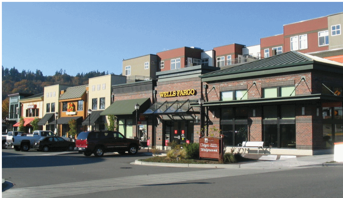
Figure C12. This development uses a variety of roof forms and heights and variations in roof textures by using metal hip roofs, different weather protection features, changing building materials and colors, and a modest amount of horizontal building modulation to reduce the overall architectural scale into smaller “storefront” components.
