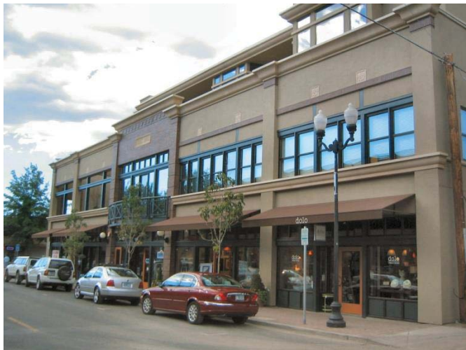
Figure C11. Example of a well-articulated building. Note how the awnings, window divisions, pilasters columns and cornice line all serve to divide up the façade into smaller segments without disrupting the unity of the overall design.
