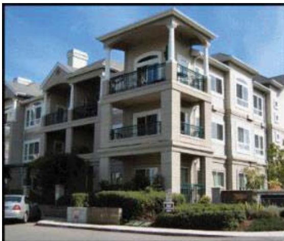
Figure C24 – A residential courtyard providing semi-private patio spaces adjacent to individual units.
