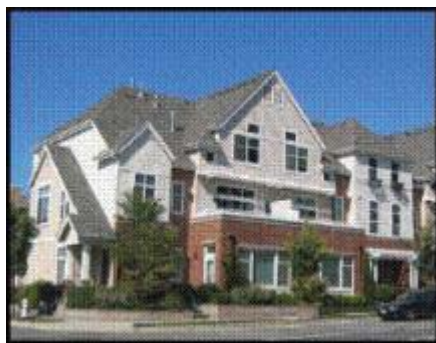
Figure B8 – Two examples of articulating a building's top, middle, and bottom by utilizing brick on the ground floor, defined window patterns and articulation treatments on upper floors, and a distinctive roofline.
