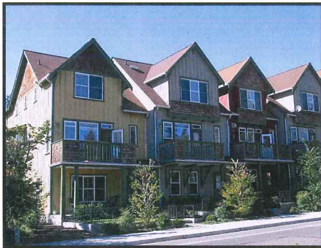
Figure 17 - Common open space for a townhouse development.
