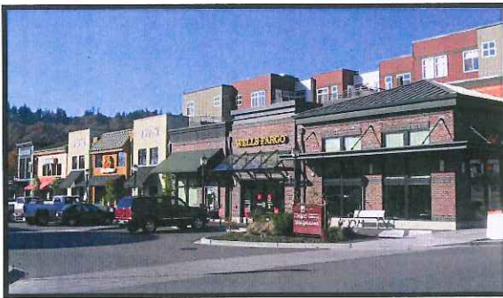
Figure 9 – This development uses a variety of roof forms and heights, different weather protection features, changing building materials and colors, and a modest amount of horizontal building modulation to reduce the overall architectural scale into smaller “storefront” components.
