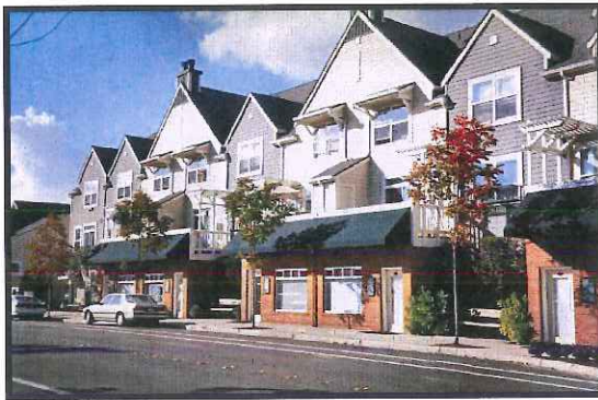
Figure 3 – This mixed-use building incorporates decks, upper level setbacks, trellises, and landscaping to meet human-scale guidelines.
