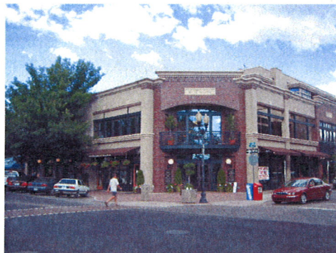
Figure 36: To emphasize its street corner location, this building uses a cropped corner, change in building materials, decorative facade elements, and a modulated roofline.
