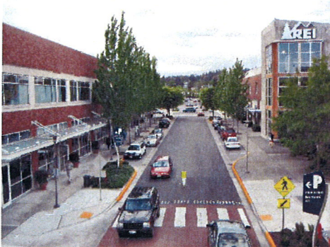
Figure 12: Redmond Town Center's internal roadways are one model. Note the on-street parking, crosswalks, wide sidewalks, street trees, signage, and pedestrian lighting.
