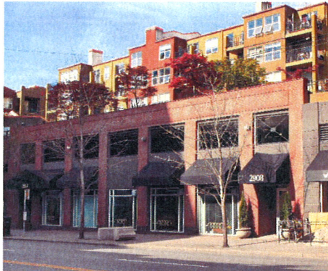
Figure 43: This building uses opening on its second level parking area to resemble windows.
