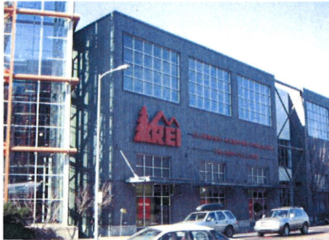
Figure 50: Example of acceptable signage for large retailers.
