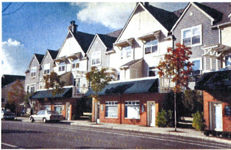
Figure 24: This mixed-use building incorporates decks, upper level setbacks, trellises, and landscaping to meet human scale guidelines.
