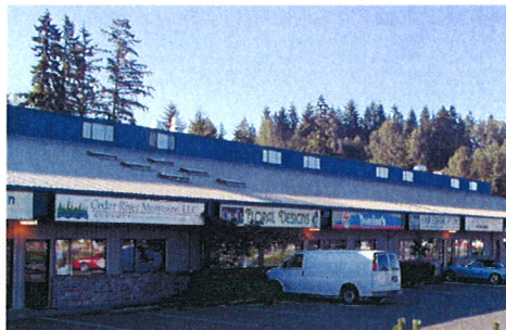
Figure 47: Back-lit signs, like these are prohibited.
