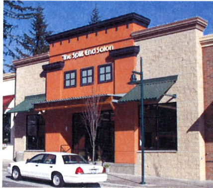
Figure 38: This storefront effectively combines EIFS and concrete block with wood trim and metal detailing.
