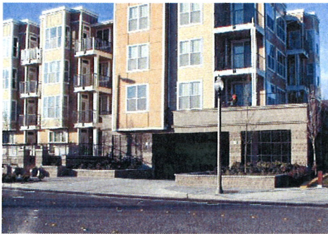
Figure 44: Design parking garages to obscure the view of parked cars. Note the landscaping that separates the garage from pedestrians.
