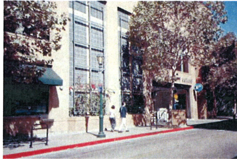
Figure 42: The side of this parking garage includes some storefront retail space (left), decorative grillwork, and a raised brick planter to enhance the pedestrian environment.
