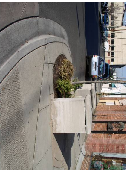
Curb bulb example at intersection.
