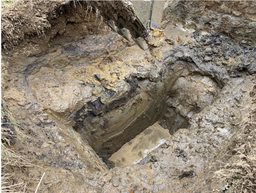
Image 1. Pilot Infiltration Test 1 excavations exposing 3.5' of dredged fill and relict topsoil overlying slightly gravelly, Marysville Sands with rapid seepage occurring at 6.8' below ground surface (BGS).
