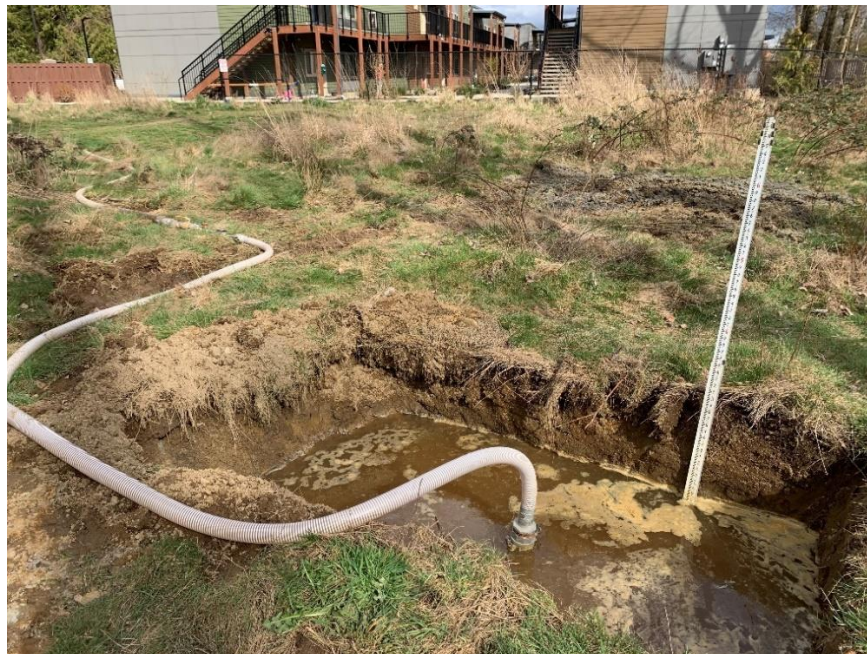
Image 2. Pilot Infiltration Test 1 set up at 2.75' BGS in the southeastern quadrant of the site within the relict topsoil unit.
