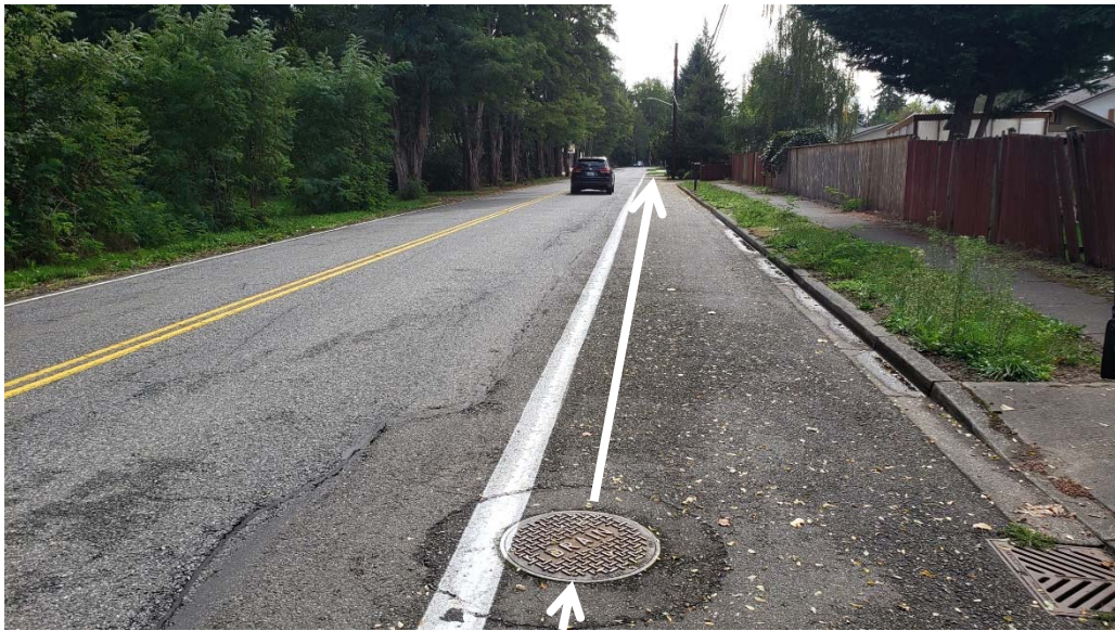
Photo #4 Looking north along 26 th Dr. SE
