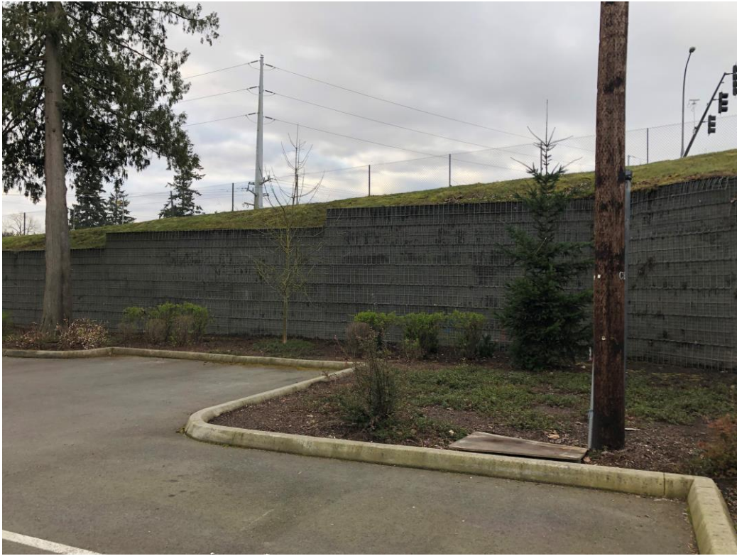
South View of 88 th Street NE Landscape Buffer
