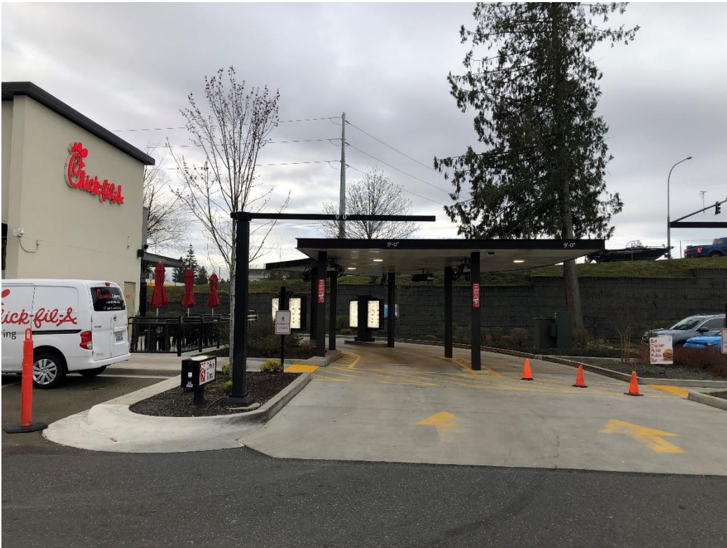
South View of Drive-thru
