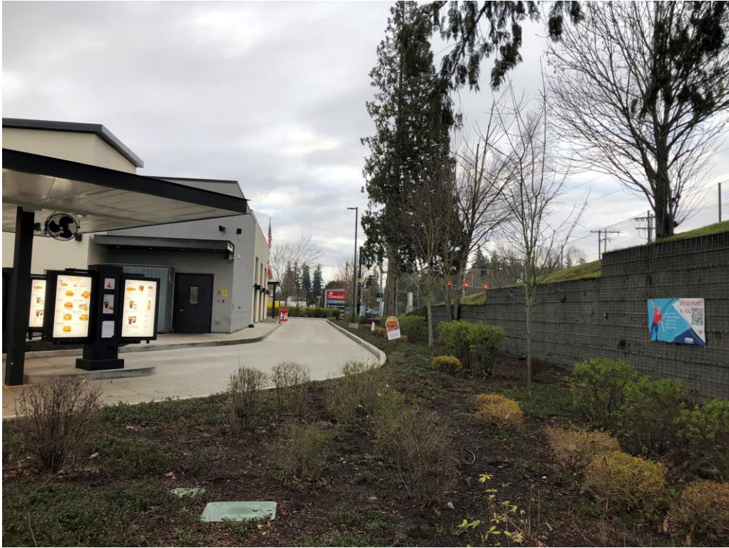
East View of 88 th Street NE Landscape Buffer
