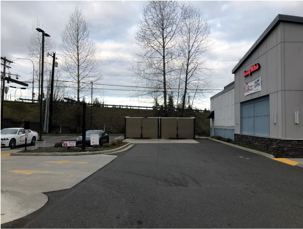
West View of Solid Waste Enclosure
