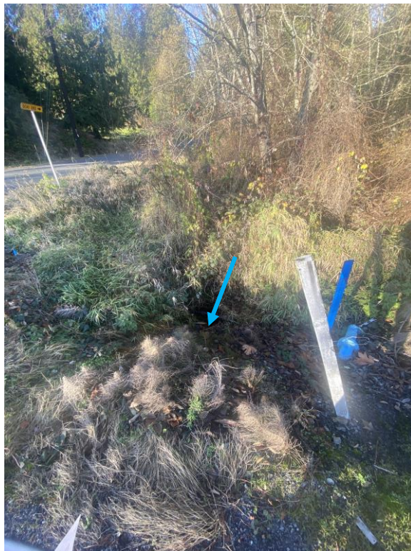
Image 4: North side of 44 th St NE, prior to King Creek crossing
