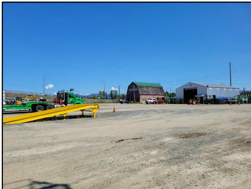
Image 1. Surface conditions of site consisted of a gravelled lot with a few buildings, facing northeast. Images 1 and 2 were taken on May 11, 2023.
