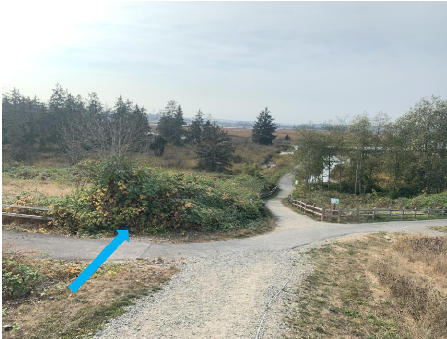
Image 3: The 8" diameter storm drain crosses under the paved pathway and outlets to a vegetated swale within the NGPA.
