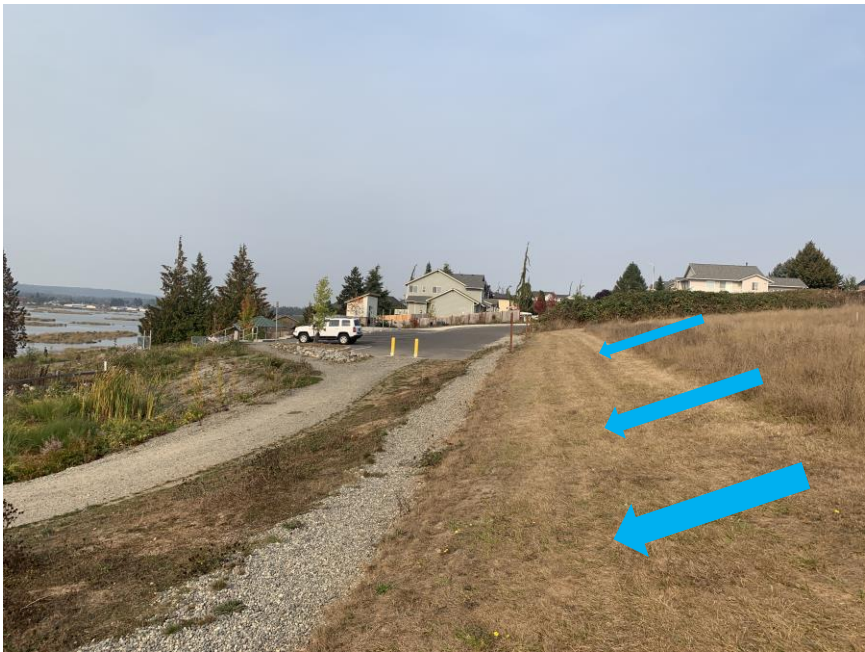
Image 2: The French drain at the east edge of Olympic View Park collects sheet flow from the Olympic Vista project site.
