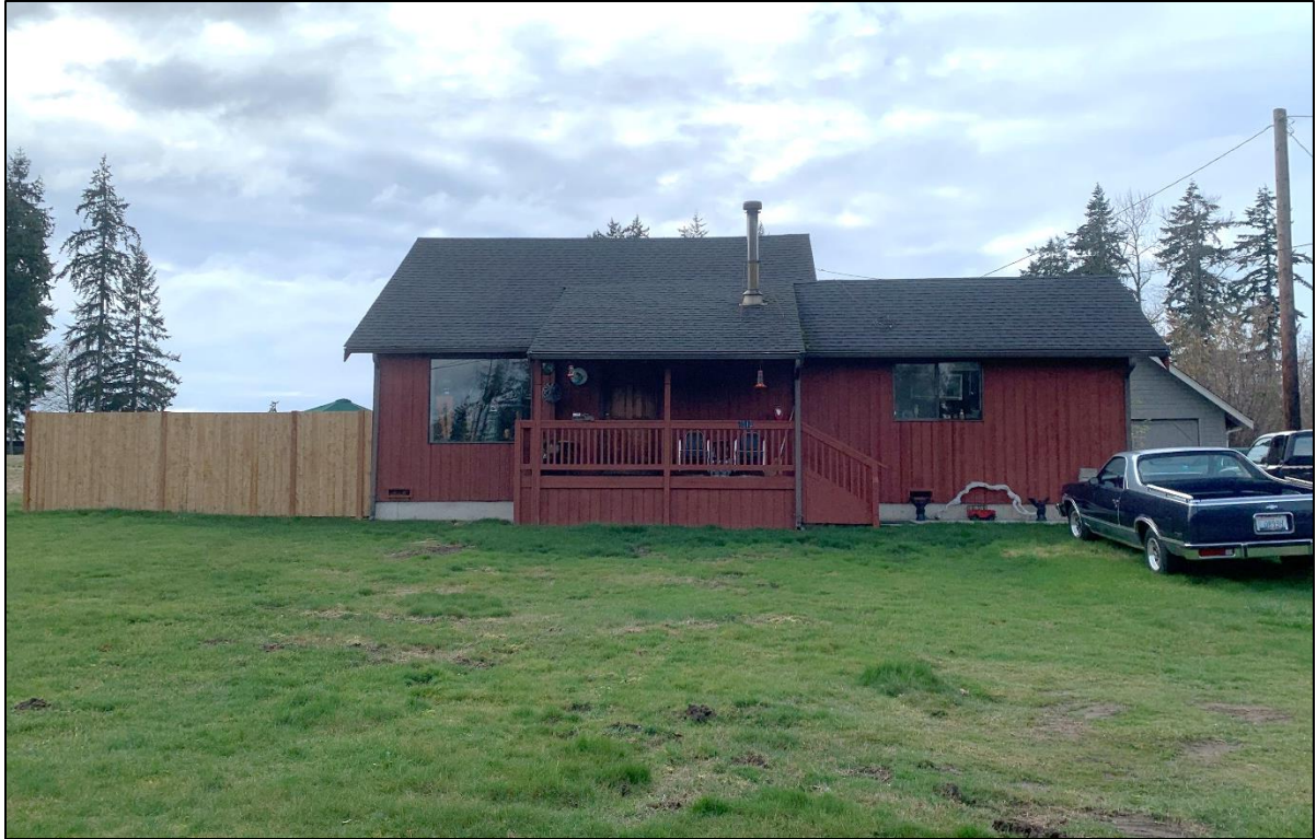
Figure 53: View west, Structure 4.
