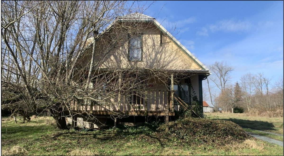
Figure 42: View west, Structure 2, Structure 1 in background.
