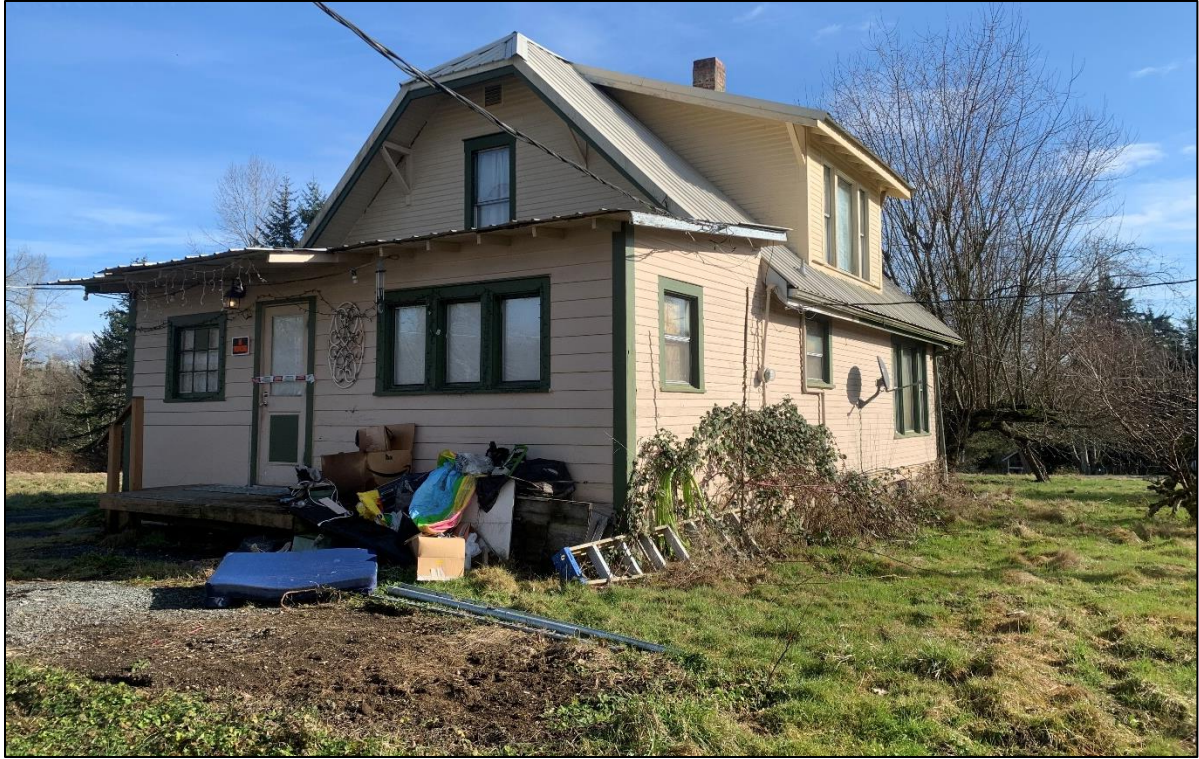
Figure 46: View northeast, Structure 2 with porch and some debris.
