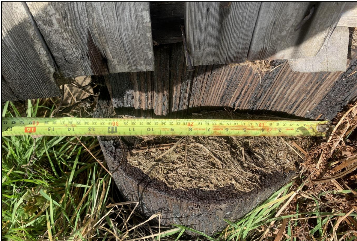
Figure 38: View west, Structure 1, detail of round foundation post near northeast corner.
