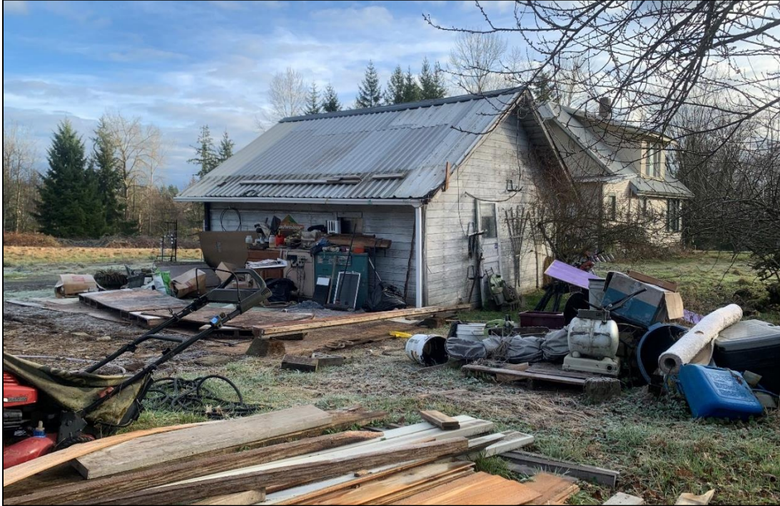
Figure 48: View northeast, Structure 3 Garage/outbuilding, with Structure 2 in the background.
