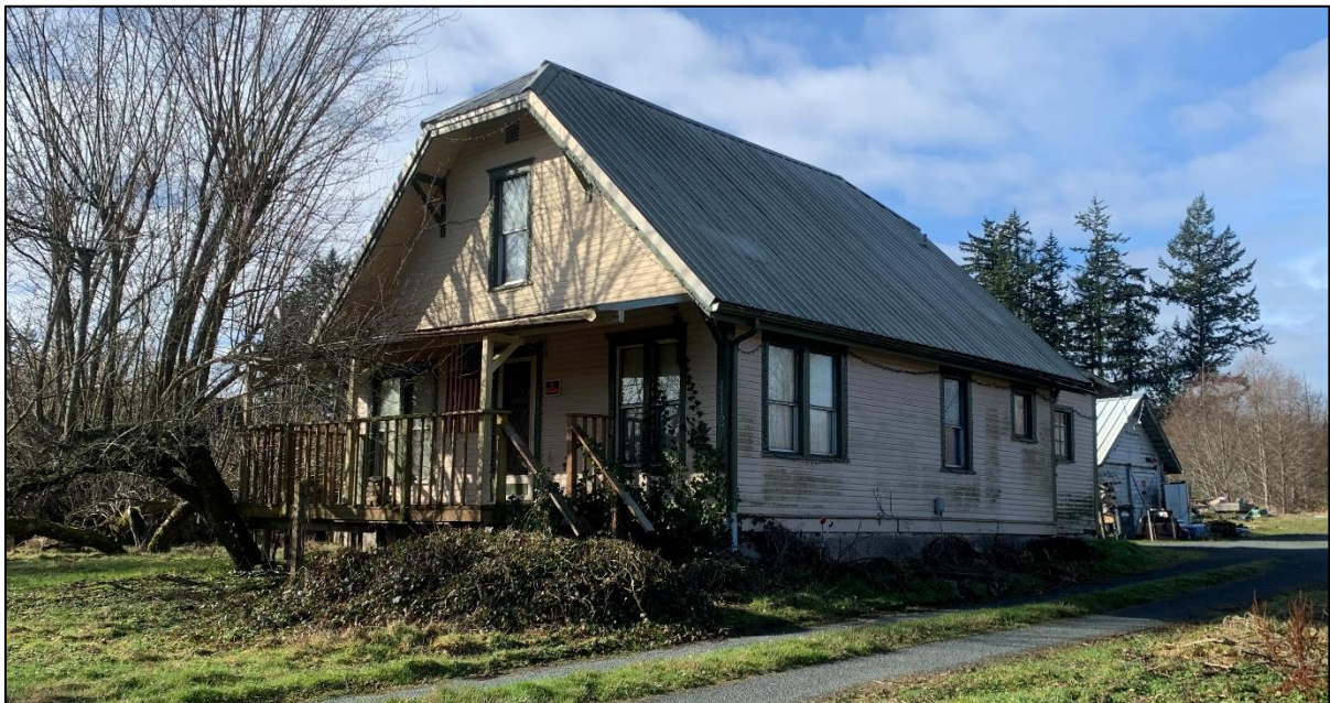
Figure 43: View southwest, Structure 2, with front porch, Structure 2 shed visible in background.
