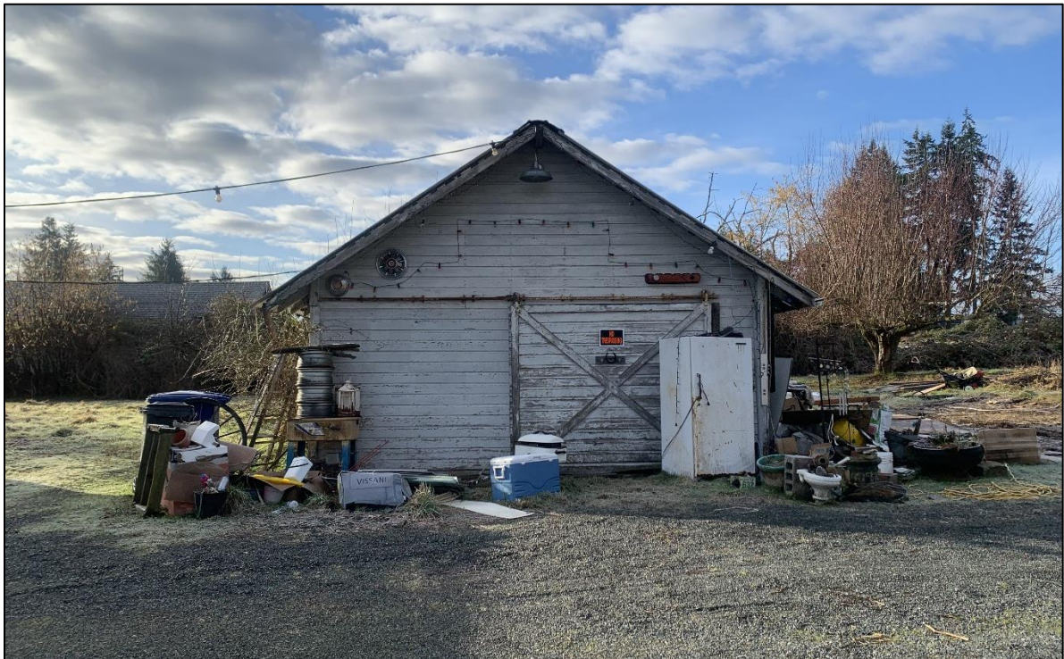
Figure 51: View south, Structure 3 Shed/outbuilding.
