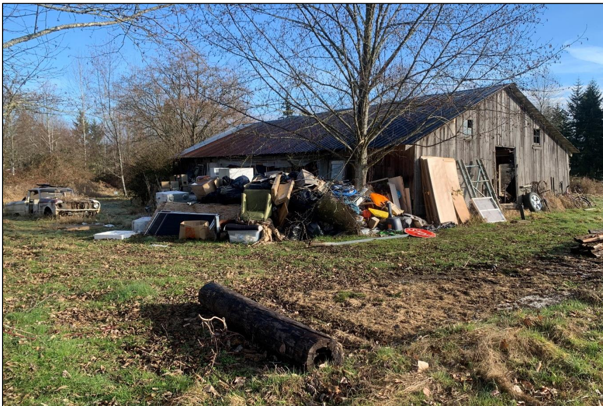
Figure 40: View northeast, Structure 1, showing residential debris along west (left) and south (right) sides.
