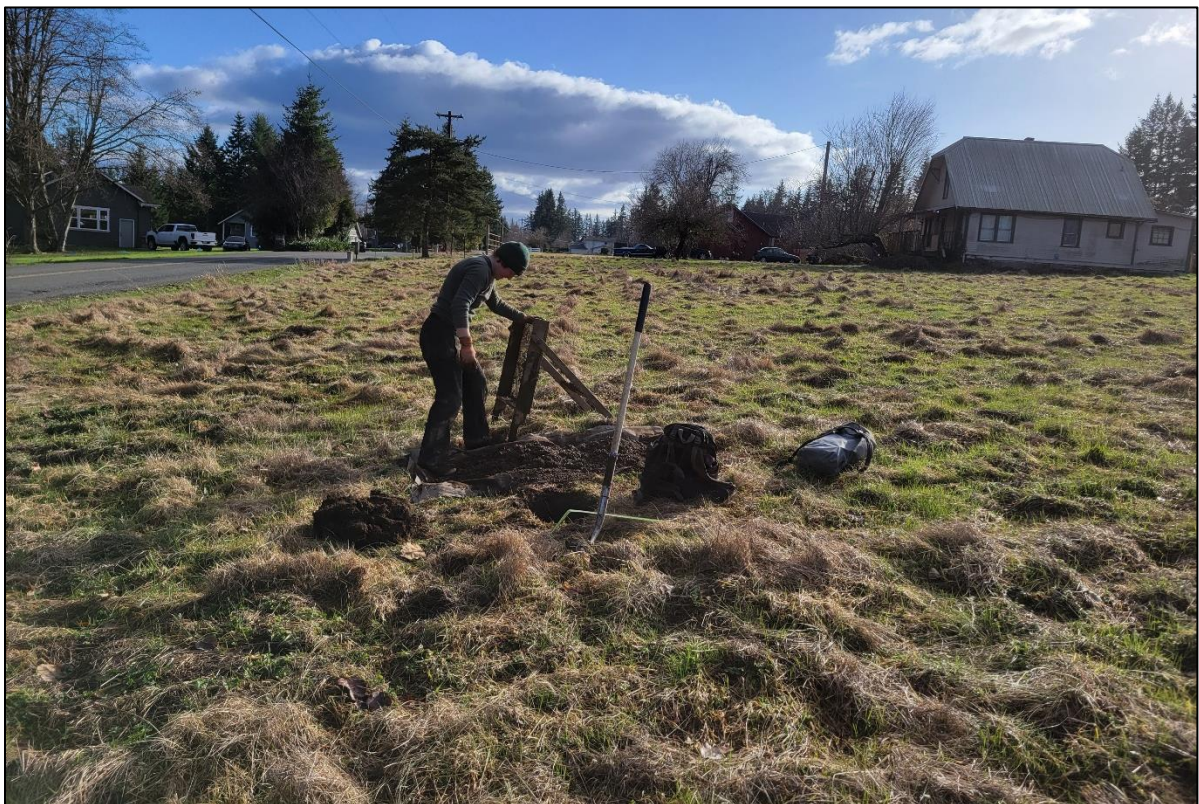
Figure 26: View west, ERCI at ST 27.
