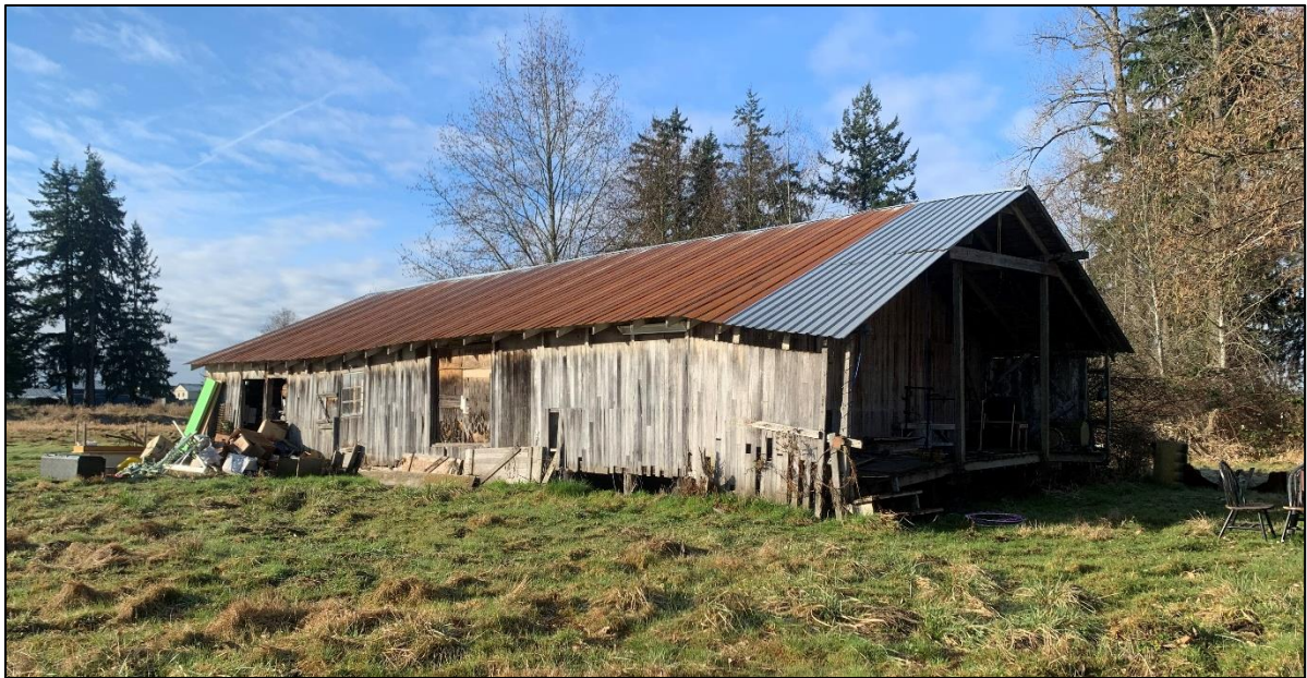
Figure 36: View southwest, Structure 1, showing east (left) and north (right) sides.
