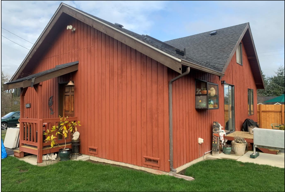
Figure 57: View northeast, Structure 4.
