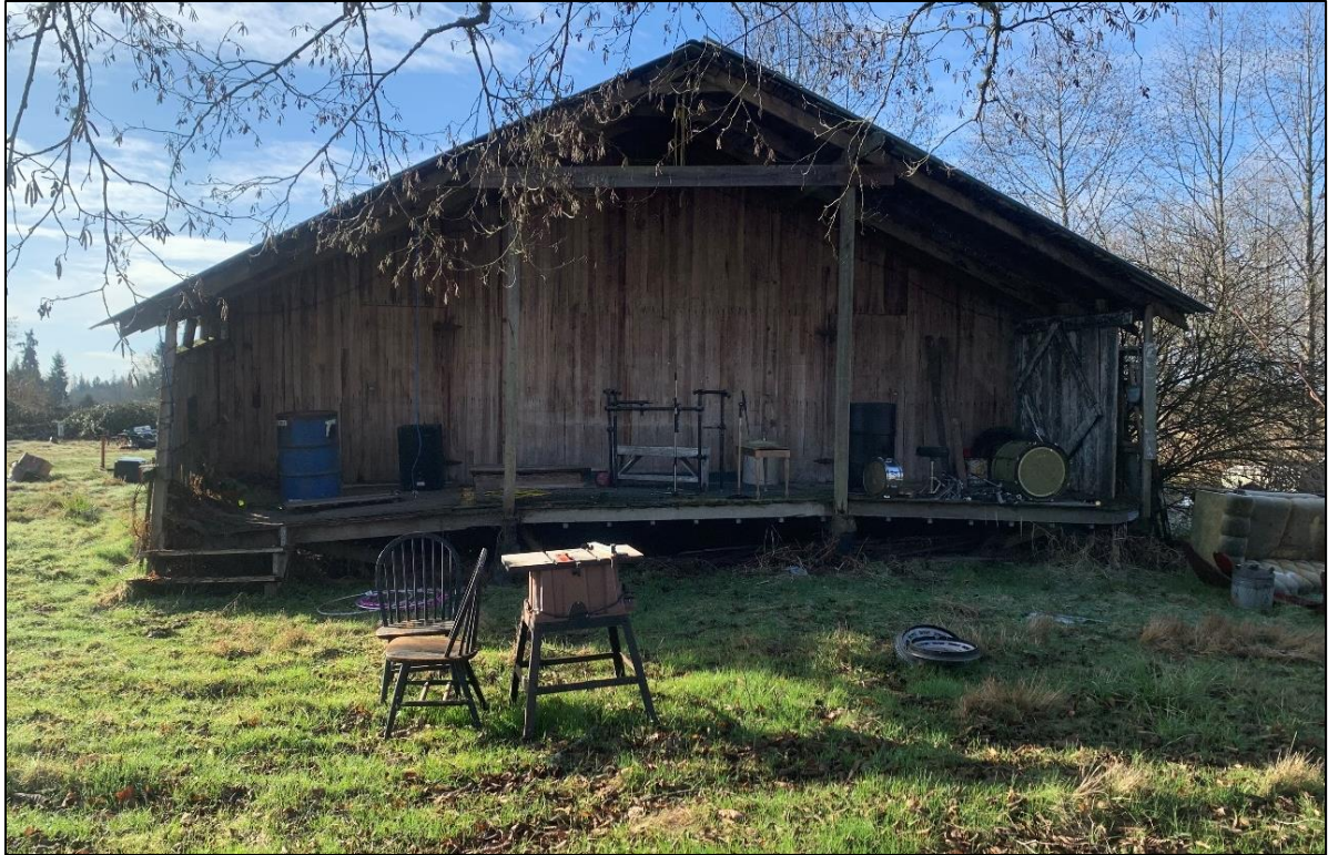
Figure 39: View south, Structure 1 with porch.
