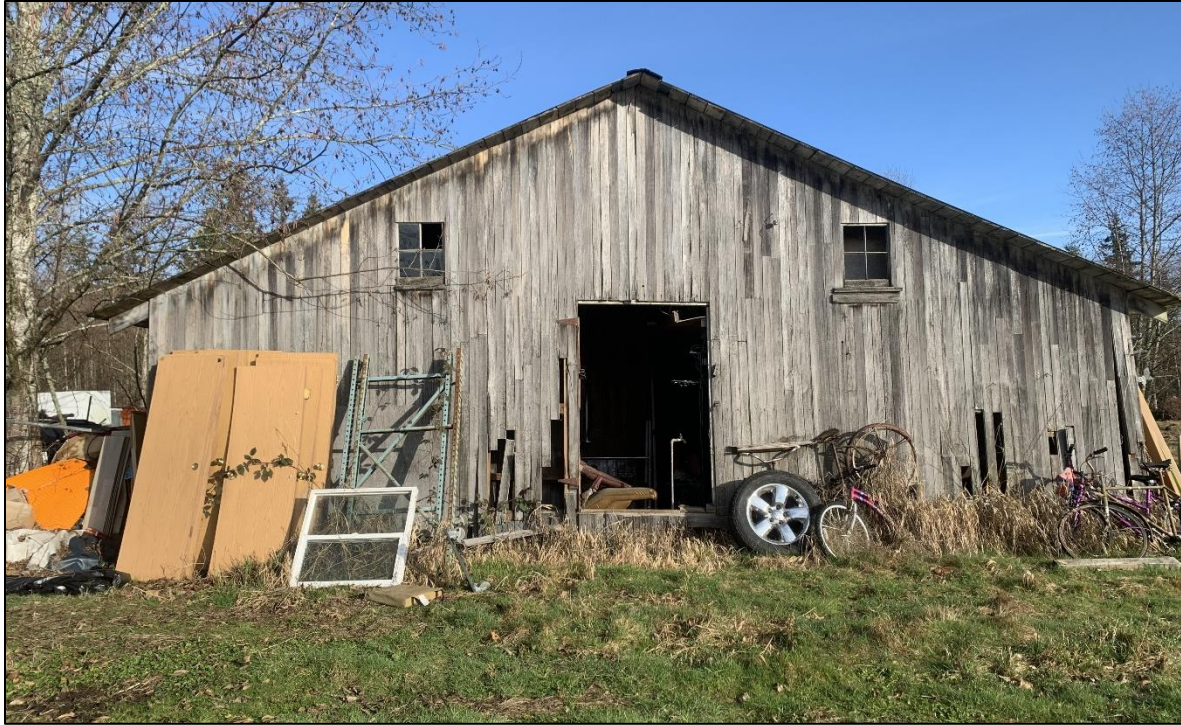
Figure 41: View north, Structure 1.
