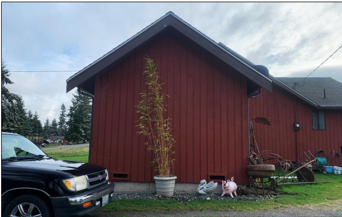
Figure 54: View south, Structure 4 addition.
