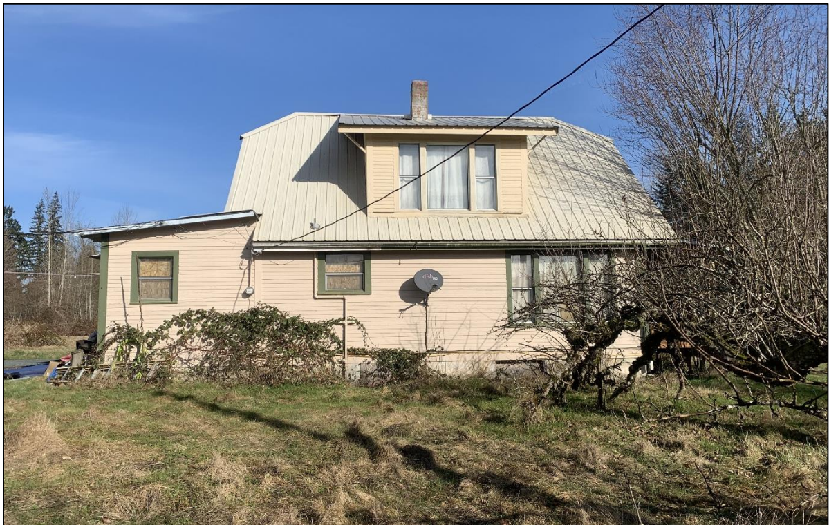
Figure 47: View north, Structure 2.
