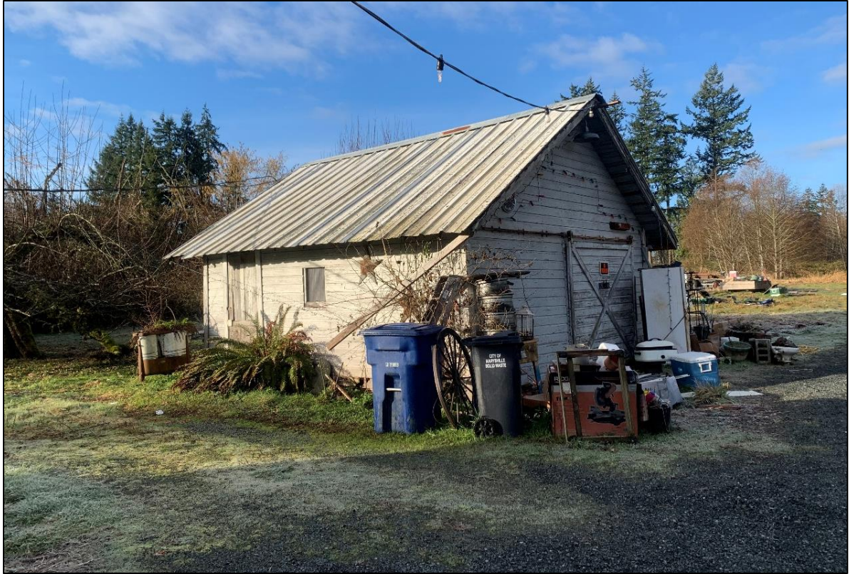
Figure 50: View southwest, Shed/outbuilding Structure 3.
