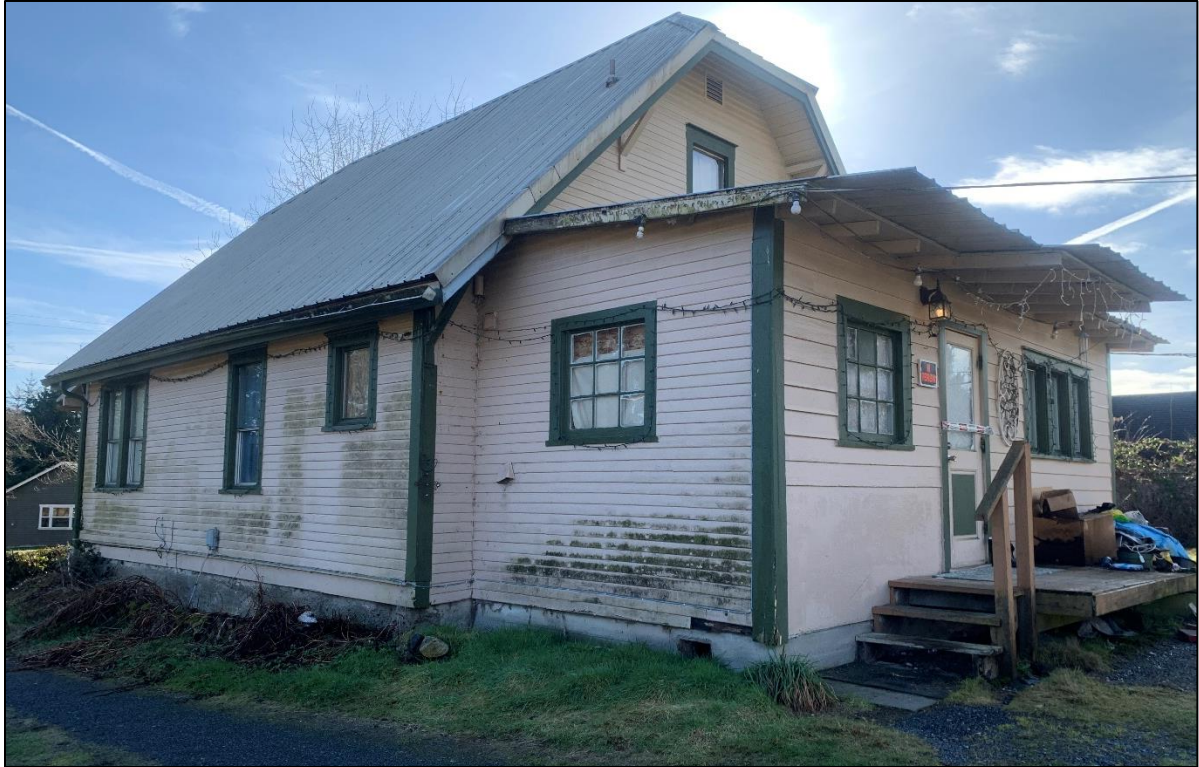
Figure 44: View southeast, Structure 2, with back porch.
