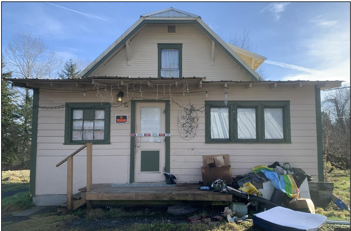
Figure 45: View east, Structure 2, west elevation, and porch.
