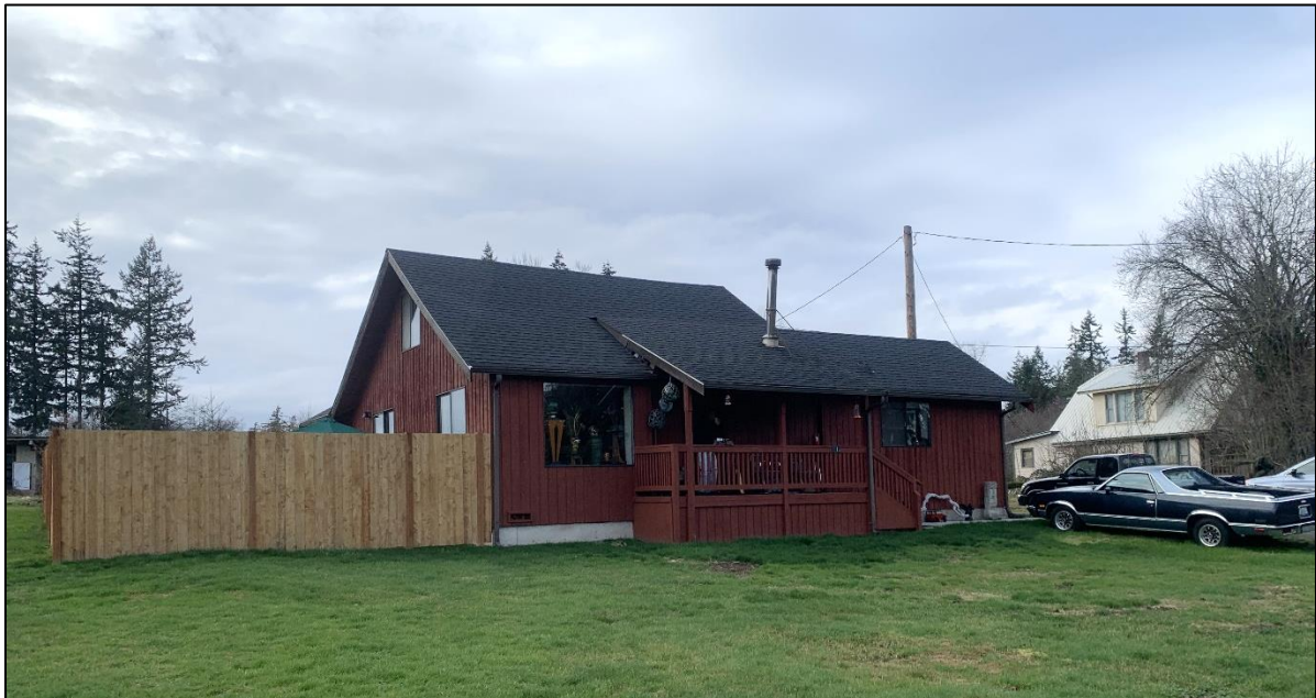
Figure 52: View northwest, Structure 4.
