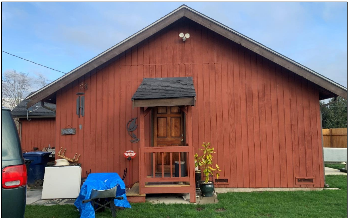
Figure 56: View east, Structure 4, west elevation.
