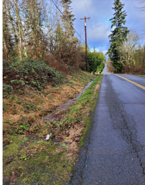
B: Drainage ditch along 87 th facing North on 87 th Ave NE
