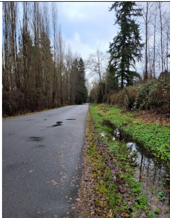
G: Densmore drainage ditch facing South
