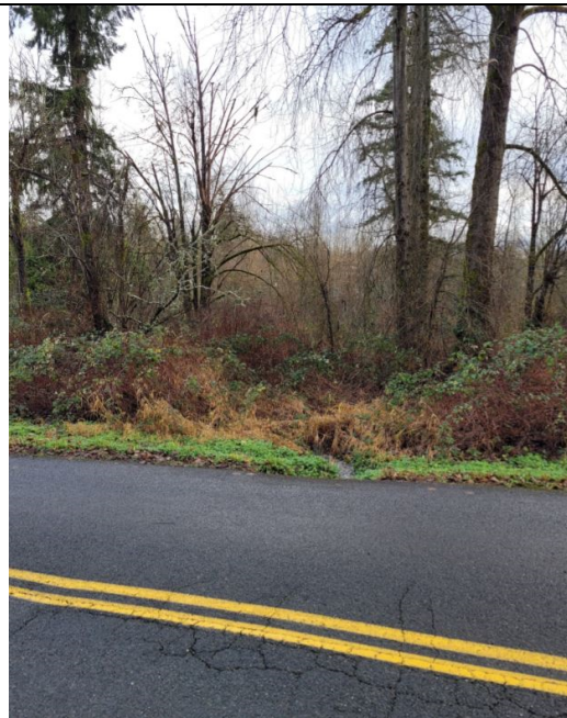
D: Culvert exit looking East over 87 th Ave NE
