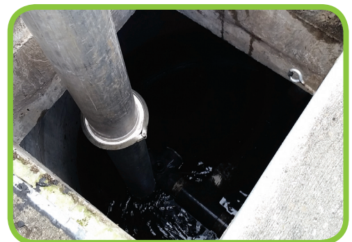
Jet Vactoring Through Access Hatch
