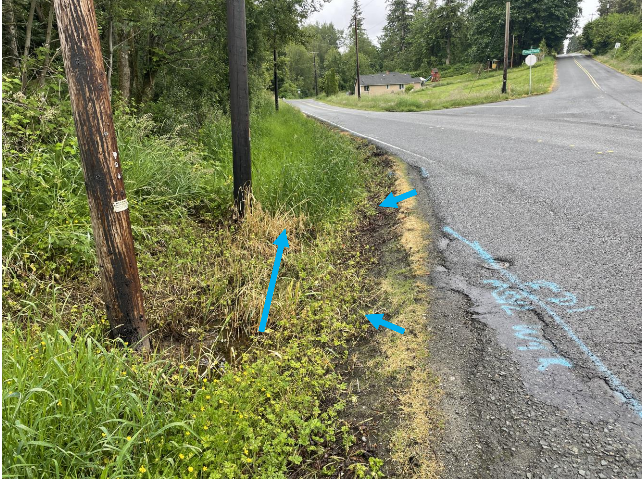
Image 5: Facing southeast from the northeast corner of the Sunnyside School Road and 87 th Ave intersection. The project site's eastern basin runoff along and near the project frontage flows south along 87 th Ave NE and discharges into the swale along the north side of Sunnyside School Road at the intersection of Sunnyside School Road and 87 th Ave. Runoff continues southeast along the Sunnyside School Road past the quarter-mile boundary of analysis until discharging into the unnamed stream tributary to Steven's Creek.
