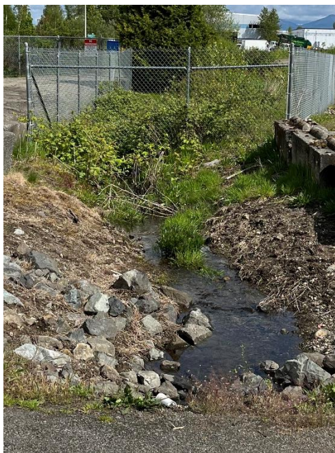
Figure 3. Regional detention pond outfall
