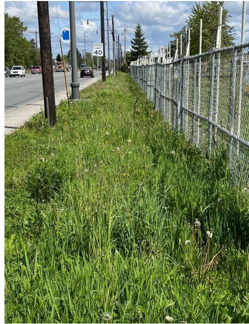
Figure 2. State Avenue channel upstream
