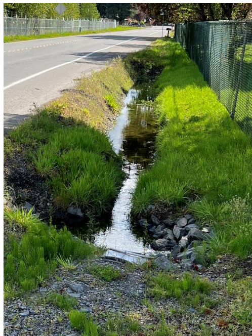
Figure 4. South of 128 th Street NE channel upstream
