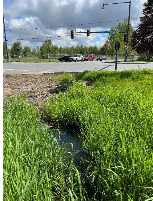
Figure 6. Inlet to channel along State Avenue
