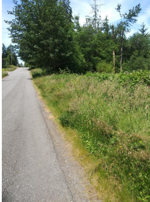
Image 1: Low point along 60 th St NE. Frontage runoff drains to this point and enters the onsite wetland before continuing north and west.
