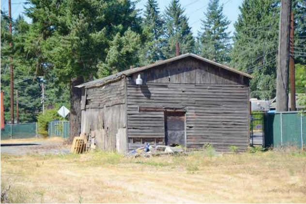
South and west sides of shed, view to the northeast.
