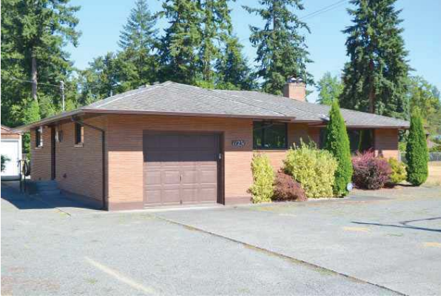
West facade, view to the east-southeast.
