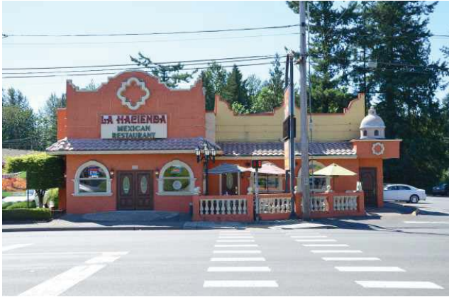
Front of building, view to the west.
