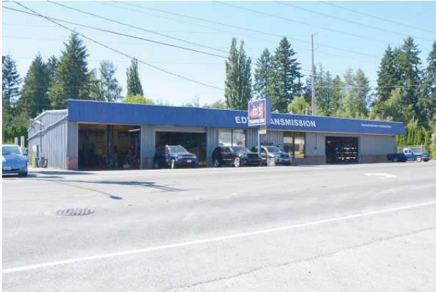
Ed's Transmission, view to the west-northwest.
