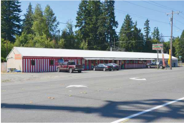
Building front, view to the west-northwest.
