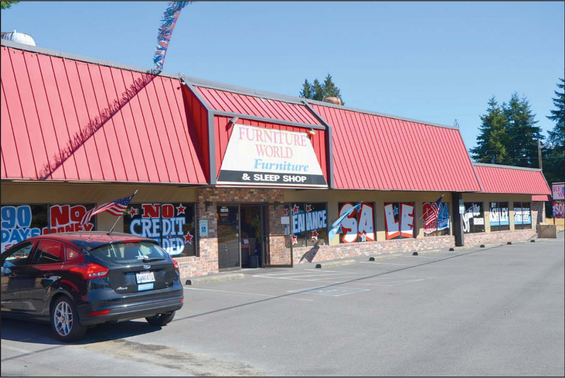
Figure 31. Furniture World (STA-17-07), south section of the building, view to the southeast.
