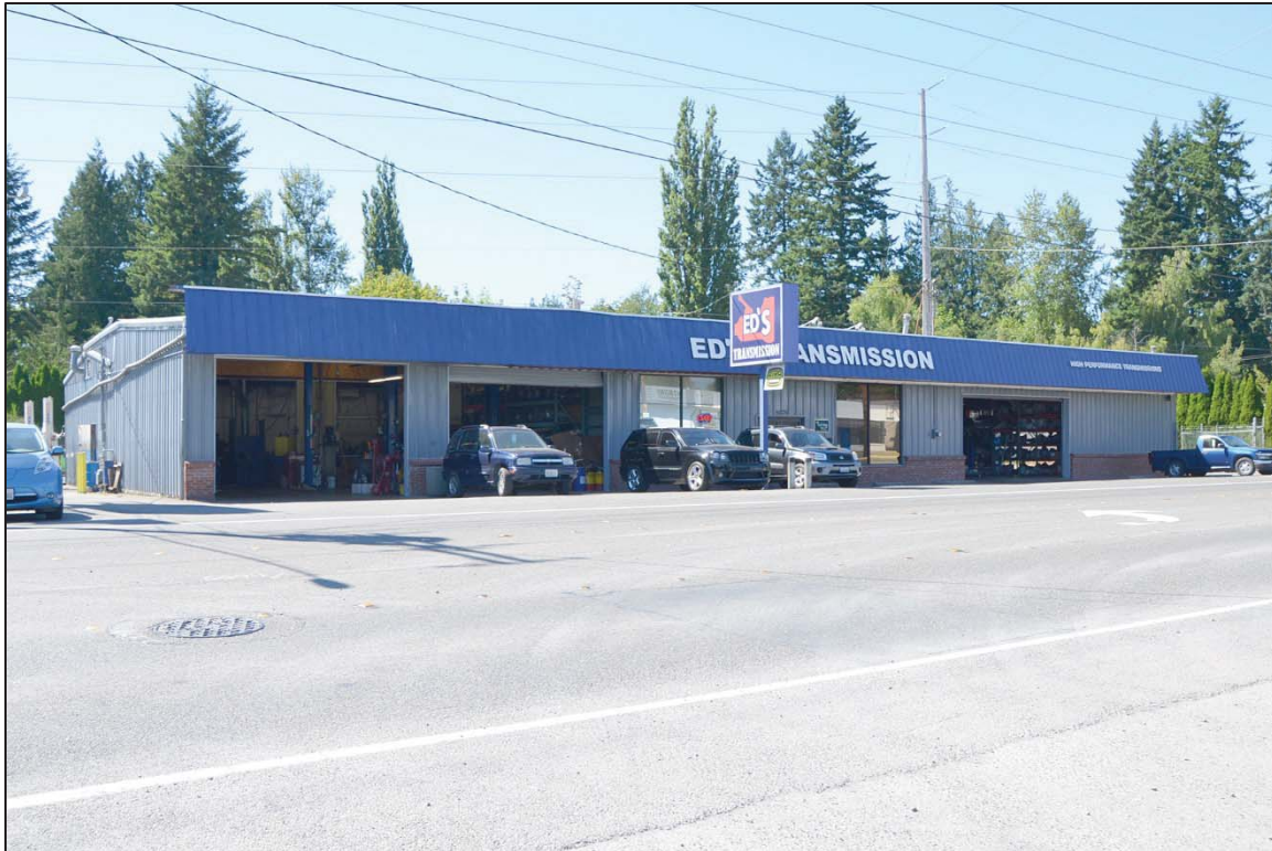
Figure 26. Ed's Transmission (STA-17-02), view to the west. The original section of the building consists of the two service bays on the south end of the building (left side of photograph).
