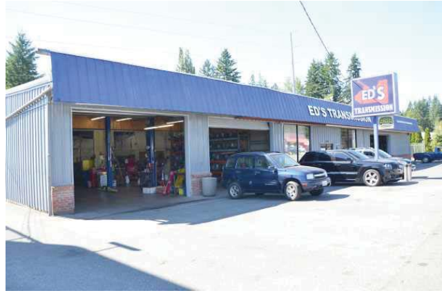
Ed's Transmission, view to the northwest.
