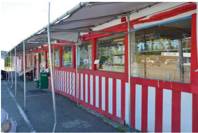
Front of store, view to the southwest.
