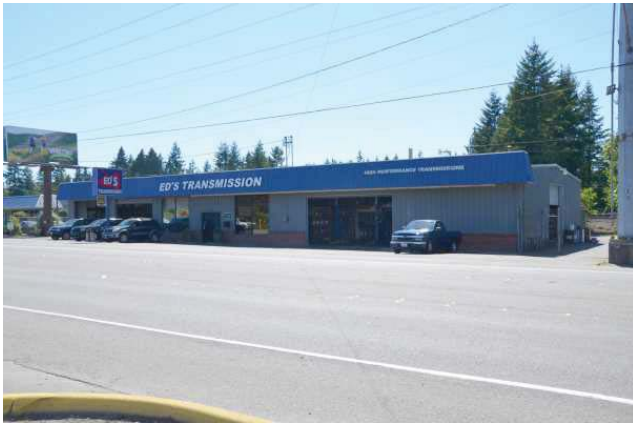
Main facade, view to the west-southwest.
