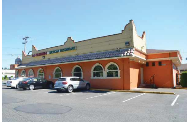
North side of building, view to the south.
