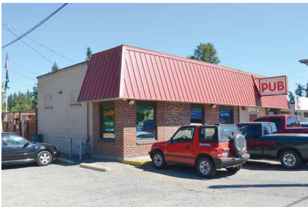
Front of building, view to the southeast.
