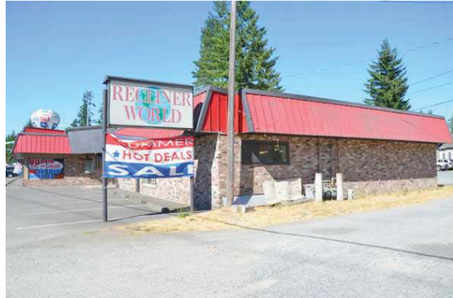
Store, view to the northeast.
