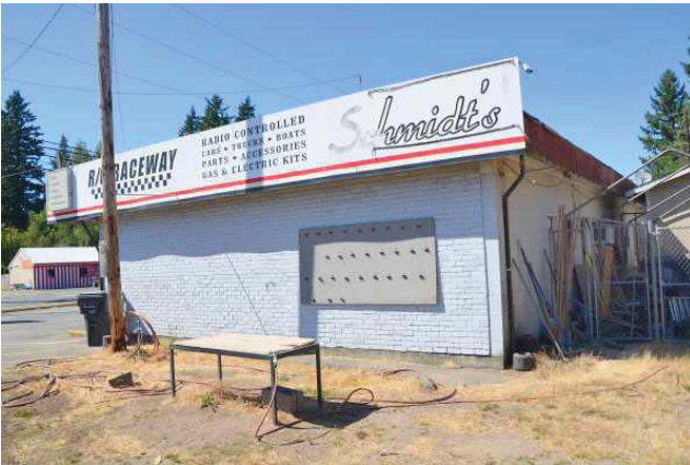
Southeast corner of the building, view to the northwest.
