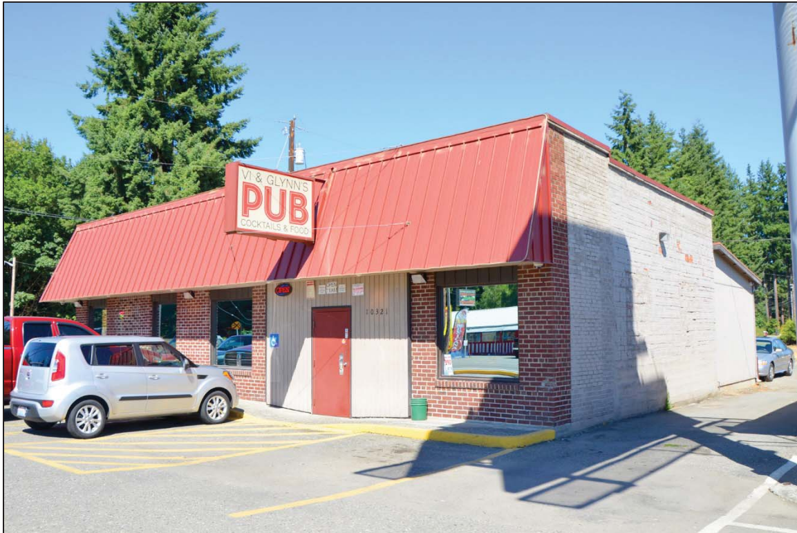
Figure 28. Vi and Glynn's Pub (STA-17-04), view to the northeast. Note alterations to entrance and addition of mansard canopy.
