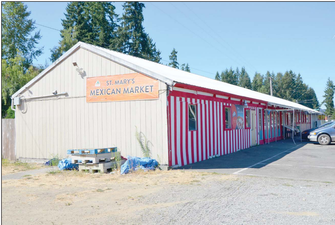
Figure 29. St. Mary's Mexican Market (STA-17-05), view to the northwest; note the addition of opaque cladding materials to convert greenhouse into a market.
