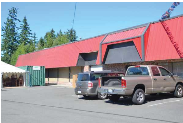
Warehouse section at north end of building; view to the northeast.
