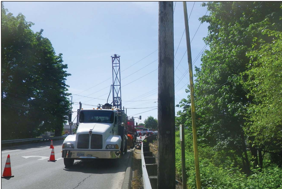
Figure 12. Borehole drilling at where State Avenue crosses over Quilceda Creek, view south.
