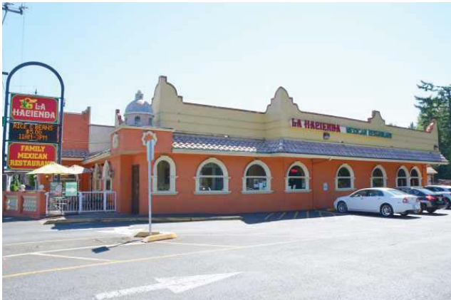
South side of building, view to the southwest.
