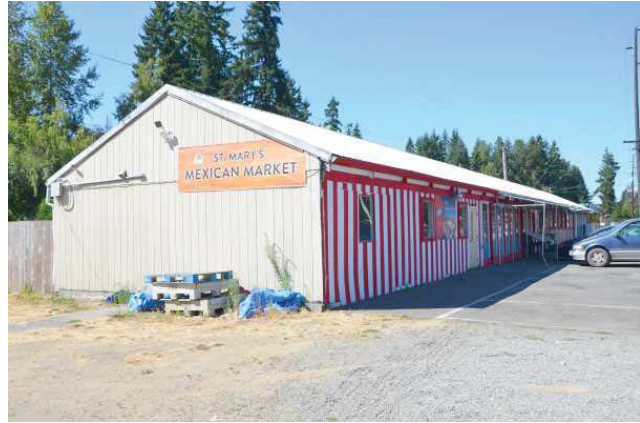
South end of building, view to the northwest.
