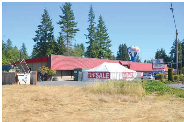
West side of building, view to the southeast.
