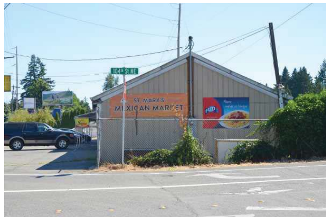
North end of building, view to the south.
