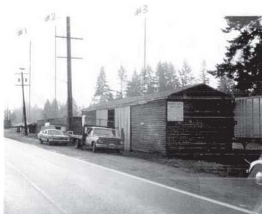
Shed, view to the southwest.
