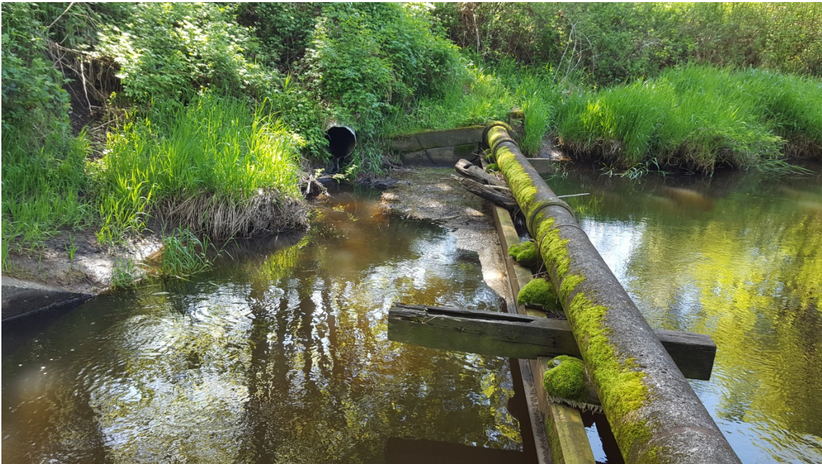
Photo 2: Quil Ceda Creek at culvert exit downstream of State Ave.
