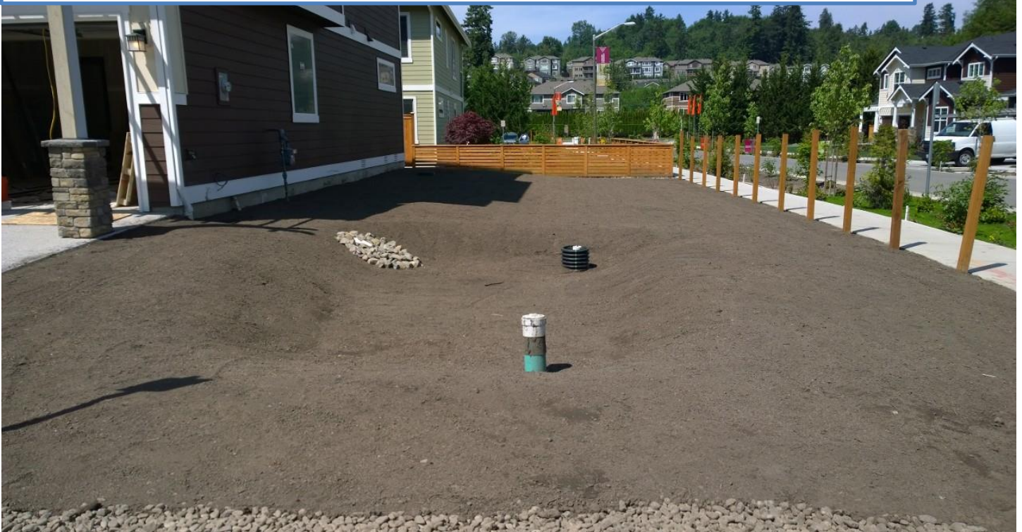
Figure 17-This shows a Biocell similar to the one above being prepared for SWM and before landscape planting.
