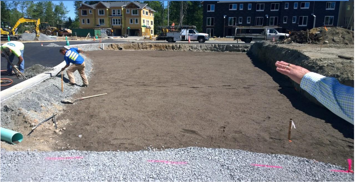
Figure 19-A biocell being prepared for Active Recreational Use. This is one of several in this Mixed Townhome-SFDU Community.
