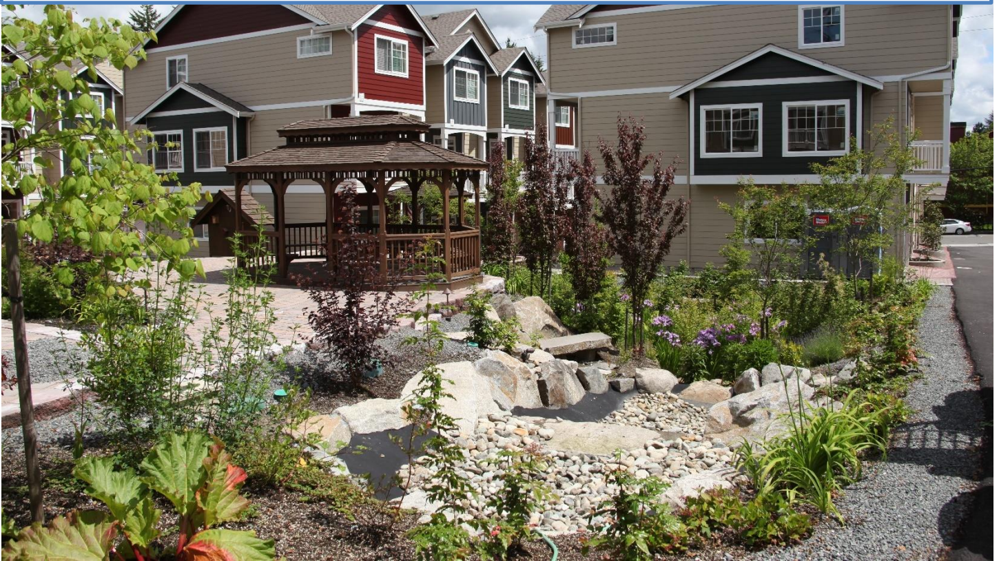
Figure 12-this is one large centralized and connected Bio-Cell that has many features for Active Recreation. We have here, pervious paths, Gazebo, Bench Swings, and arched bridge. The rock pond below has a storage tank beneath that catches stormwater for late irrigation. Birdhouses are numerous and spread out through the open space to attract and provide for wildlife.
