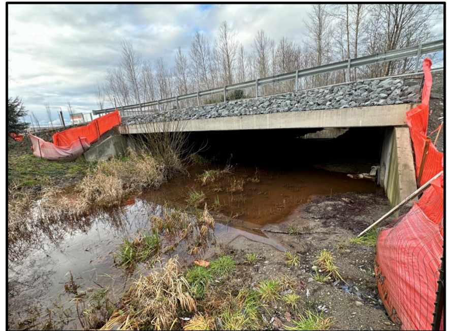
PHOTO 8: 156th Street NE extension over Hayho Creek.
