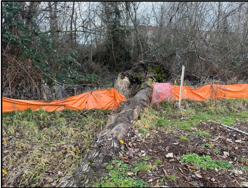
PHOTO 5: Large woody material placement in the southern buffer enhancement area.
