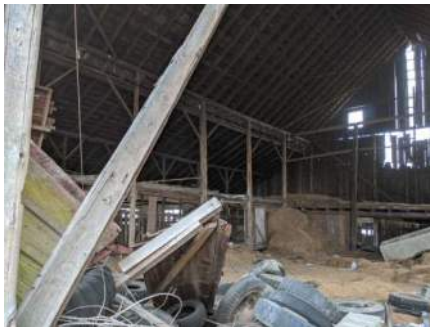
Internal, north half of main structure
