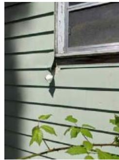
south elevation, close up of siding
