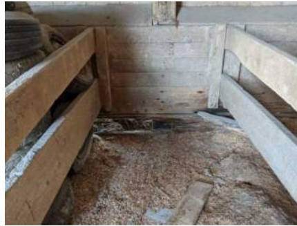
north elevation, internal, close up of foundation and stall addition
