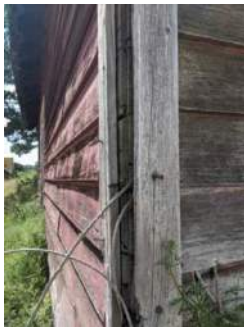
south elevation, close up of siding
