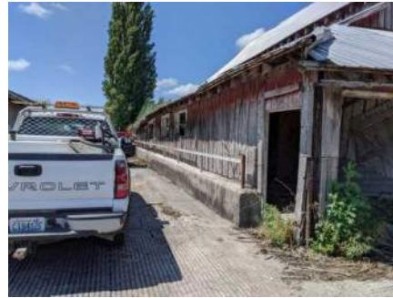
cement loading ramp, south elevation of Barn 2
