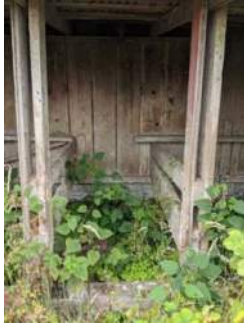
stall in northern lean-to addition
