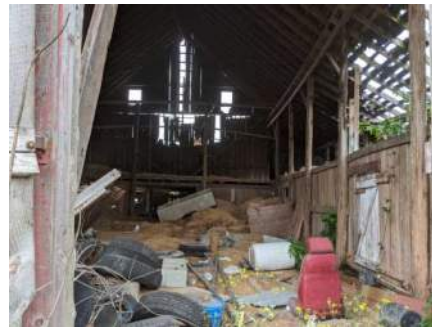
Internal, center of main structure, east elevation
