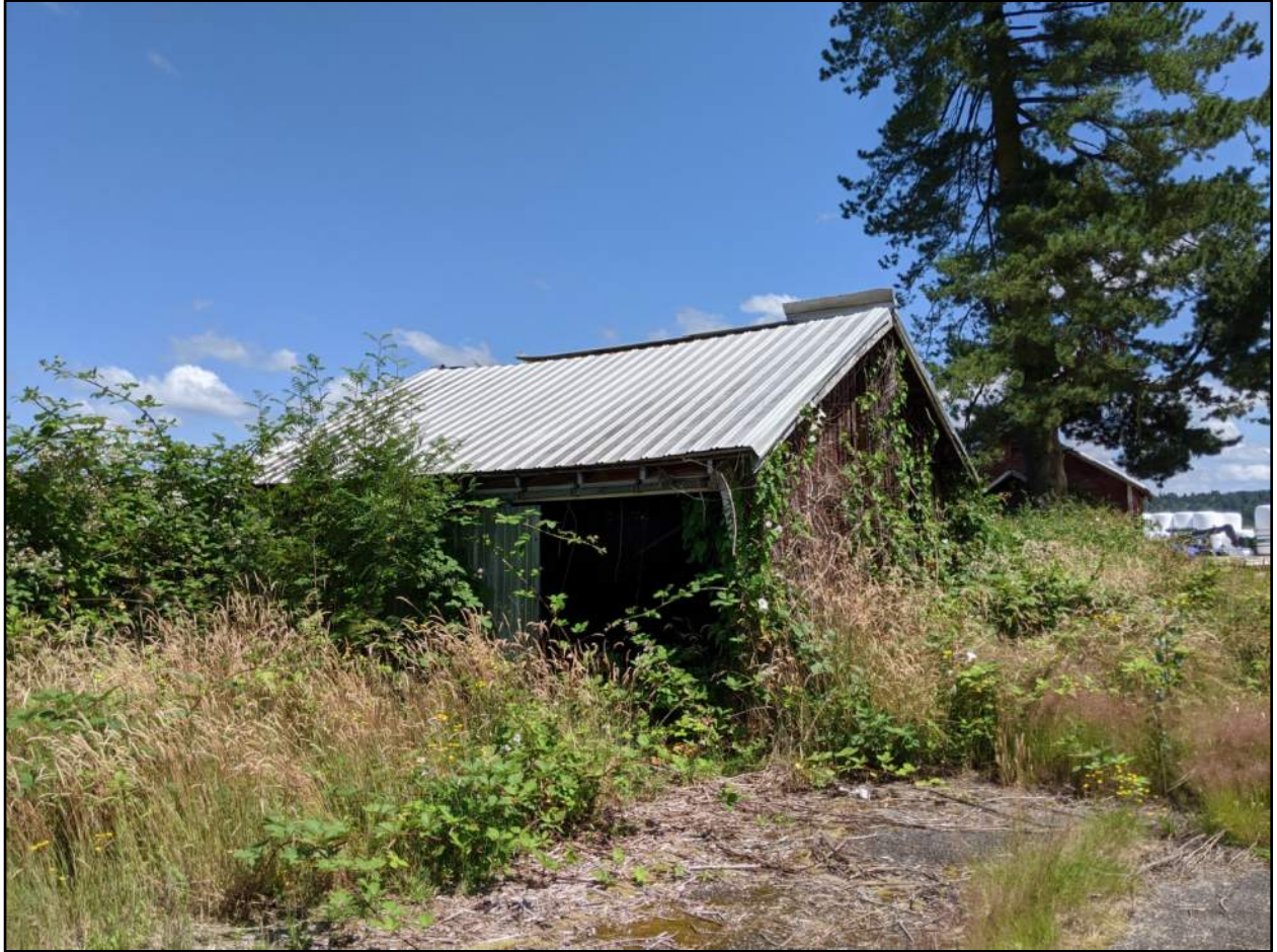
Figure 16. Garage-like structure at 16329 51st Avenue NE. Image of west and south elevations, view to the east northeast.
