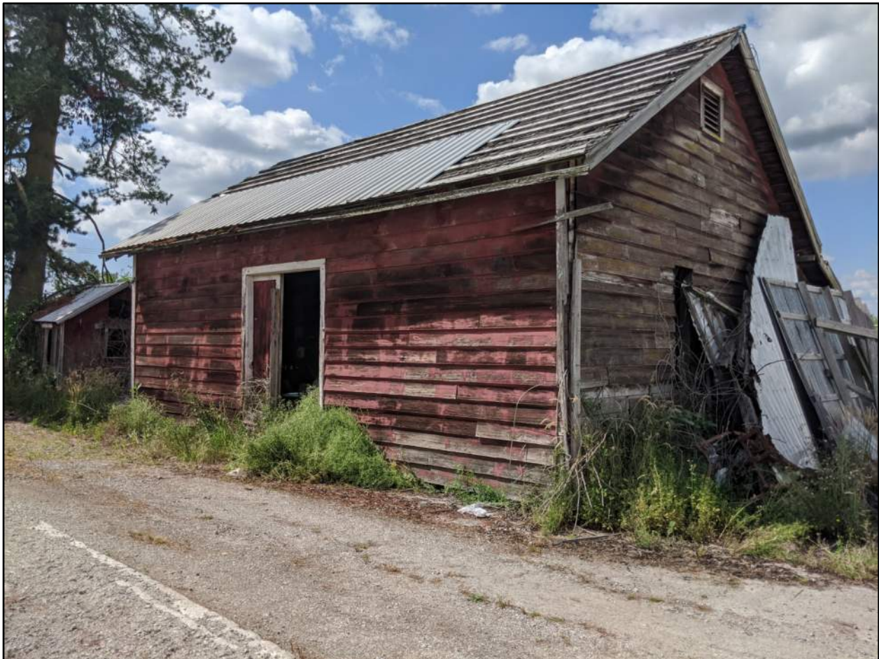
Figure 13. Outbuilding 2 (DAHP Property 722502) at 16329 51st Avenue NE. Image of south and east elevation, view to the northwest.
