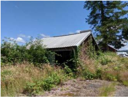
west and south elevations
