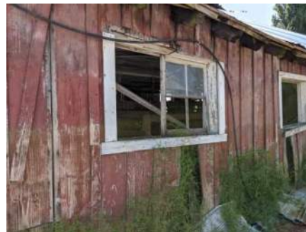
north elevation, close up of fenestration
