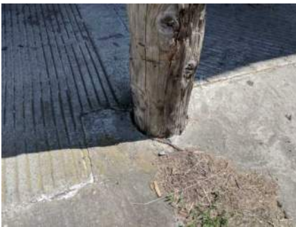
west elevation, close up of post
