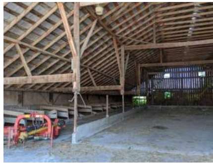
north and east elevation, internal, altered floor and construction
