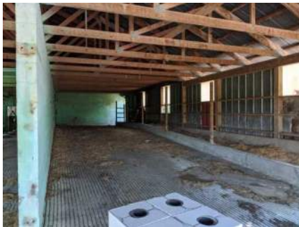
Livestock ramp, internal room
