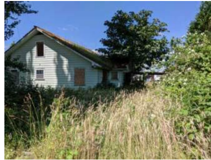
south and east elevations
