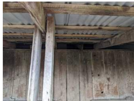
underside of roof, juncture of central and northern additions
