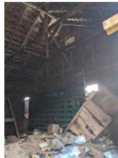
east elevation, interior
