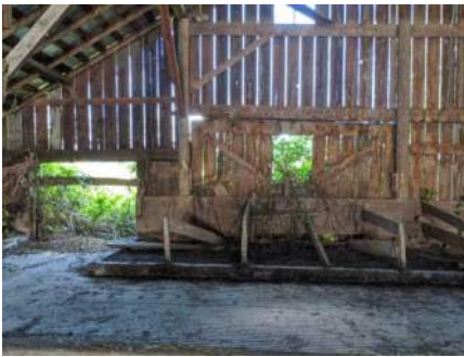
east elevation, internal, north half
