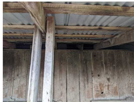
underside of roof, juncture of central and northern additions
