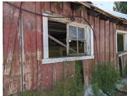
north elevation, close up of fenestration
