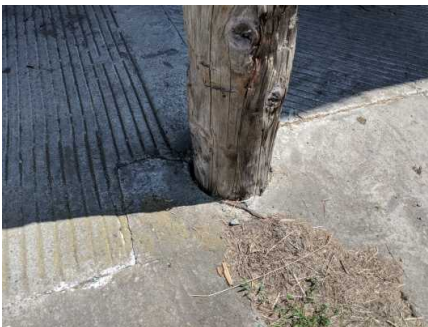
west elevation, close up of post
