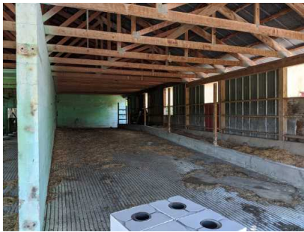
Livestock ramp, internal room
