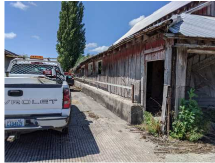
cement loading ramp, south elevation of Barn 2
