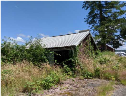
west and south elevations
