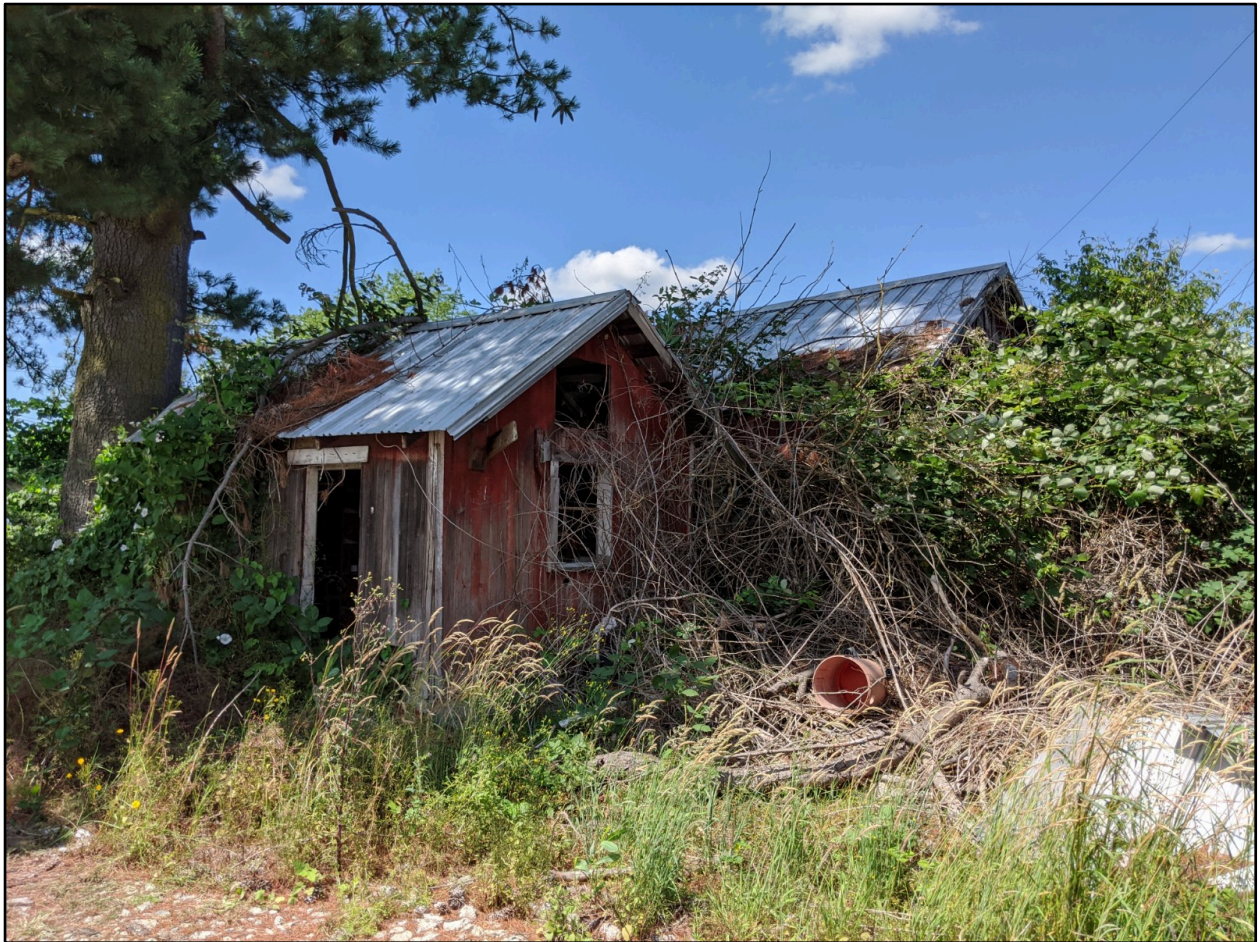
Figure 15. Shed and Outbuilding 3 (DAHP Property #722503) at 16329 51st Avenue NE. Image of south and east elevations of shed (foreground) and southeast corner of Outbuilding 3 (background), view to the northwest.
