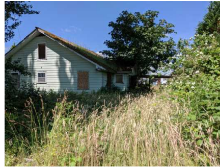
south and east elevations
