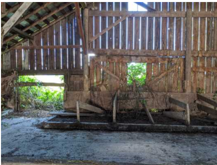
east elevation, internal, north half
