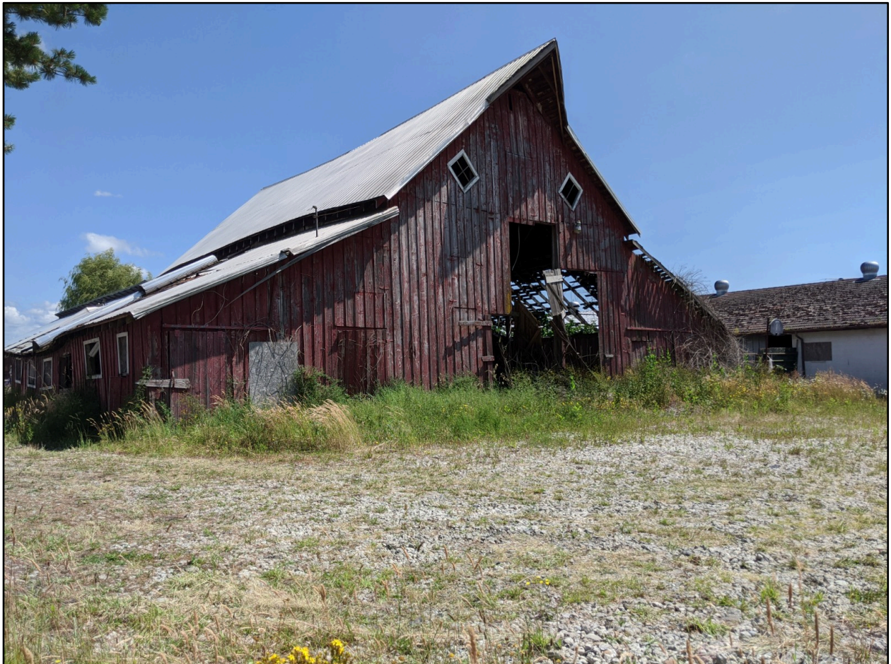
Figure 11. Barn 2 (DAHP Property #722500) at 16329 51st Avenue NE. Image of west and north elevations, view to the southeast.
