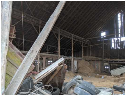
Internal, north half of main structure
