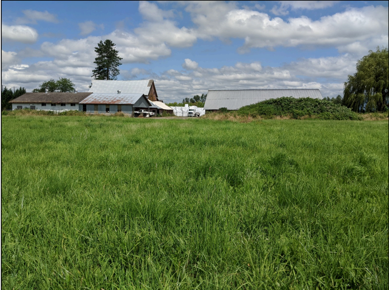
Figure 7. Overview of farm complex structures Barns 1 and 2 and Outbuilding 1. View to the north, taken from Probe 33.
