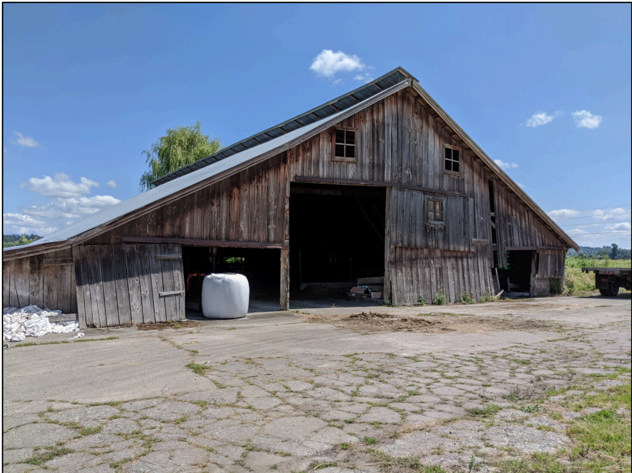
Figure 10. Barn 1 (DAHP Property #722499) at 16329 51 st Avenue NE. Image of western elevation, view to the southeast.
