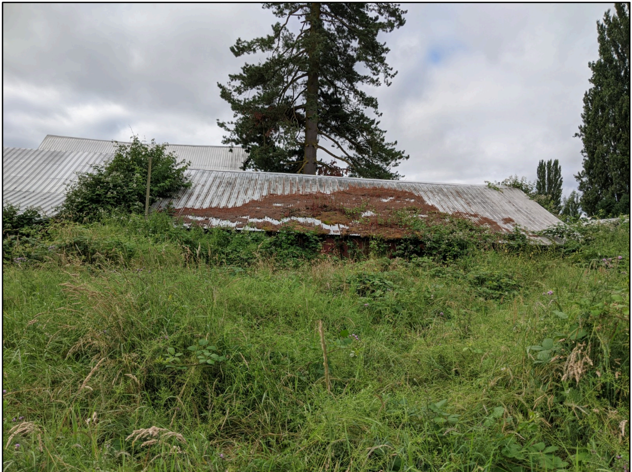
Figure 14. Outbuilding 3 (DAHP Property # 722503) at 16329 51 st Avenue NE. Image of north elevation, view to the south. Trees or tall brush to left divide Outbuildings 3 and 2 (DAHP Property # 722502).
