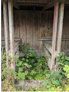
stall in northern lean-to addition
