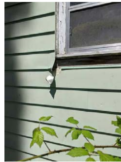
south elevation, close up of siding
