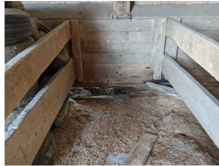
north elevation, internal, close up of foundation and stall addition
