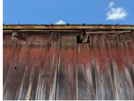
south elevation, close up
