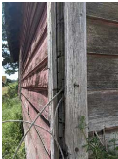
south elevation, close up of siding
