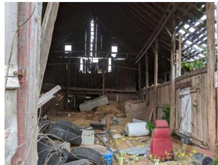
Internal, center of main structure, east elevation
