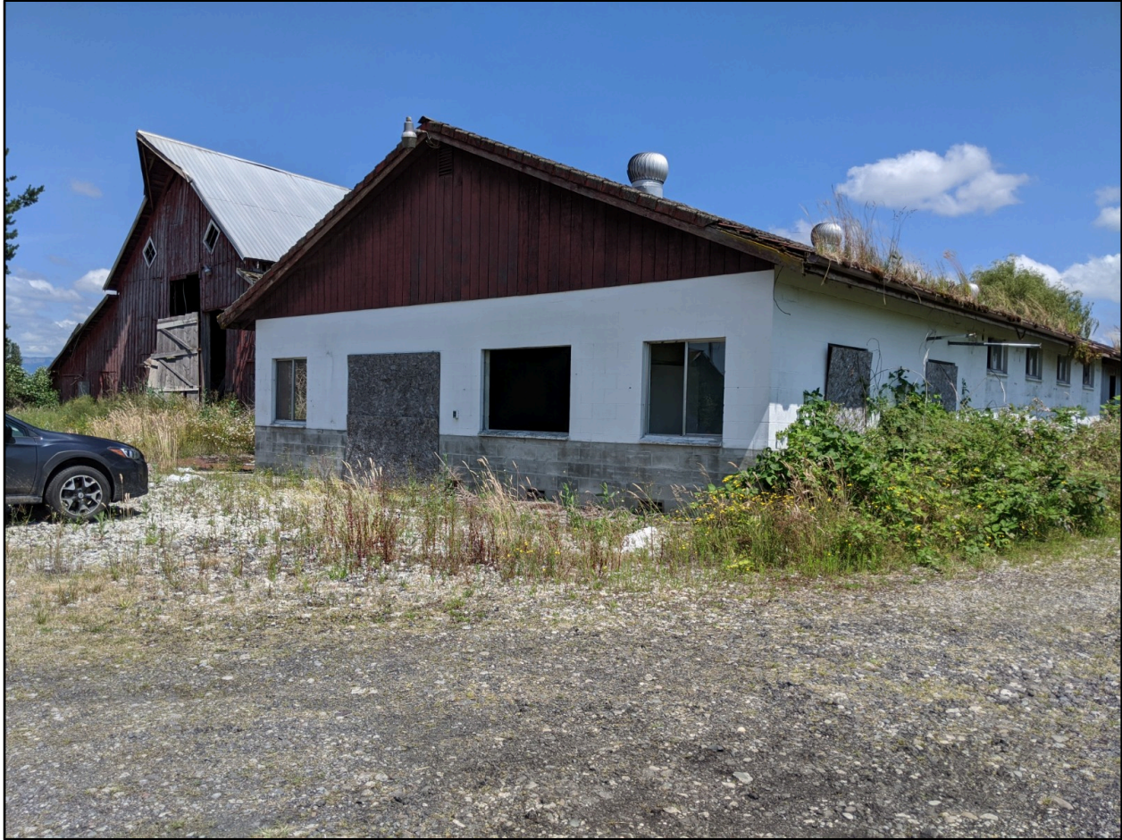
Figure 12. Outbuilding 1 (DAHP Property #722501) at 16329 51st Avenue NE. Image of west and south elevations, view to the northeast.
