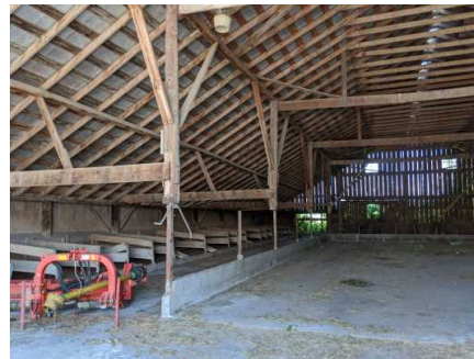
north and east elevation, internal, altered floor and construction
