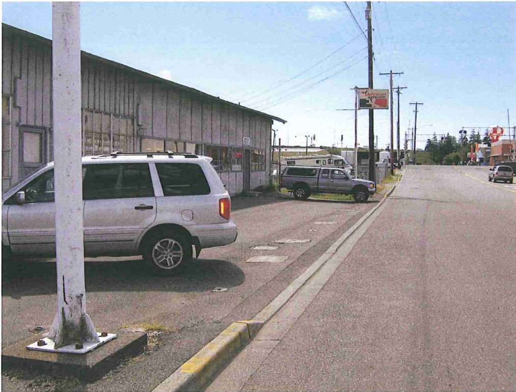
Photograph of the northern portion of the subject site and boat supply store located along First Street. Viewing to the west.
