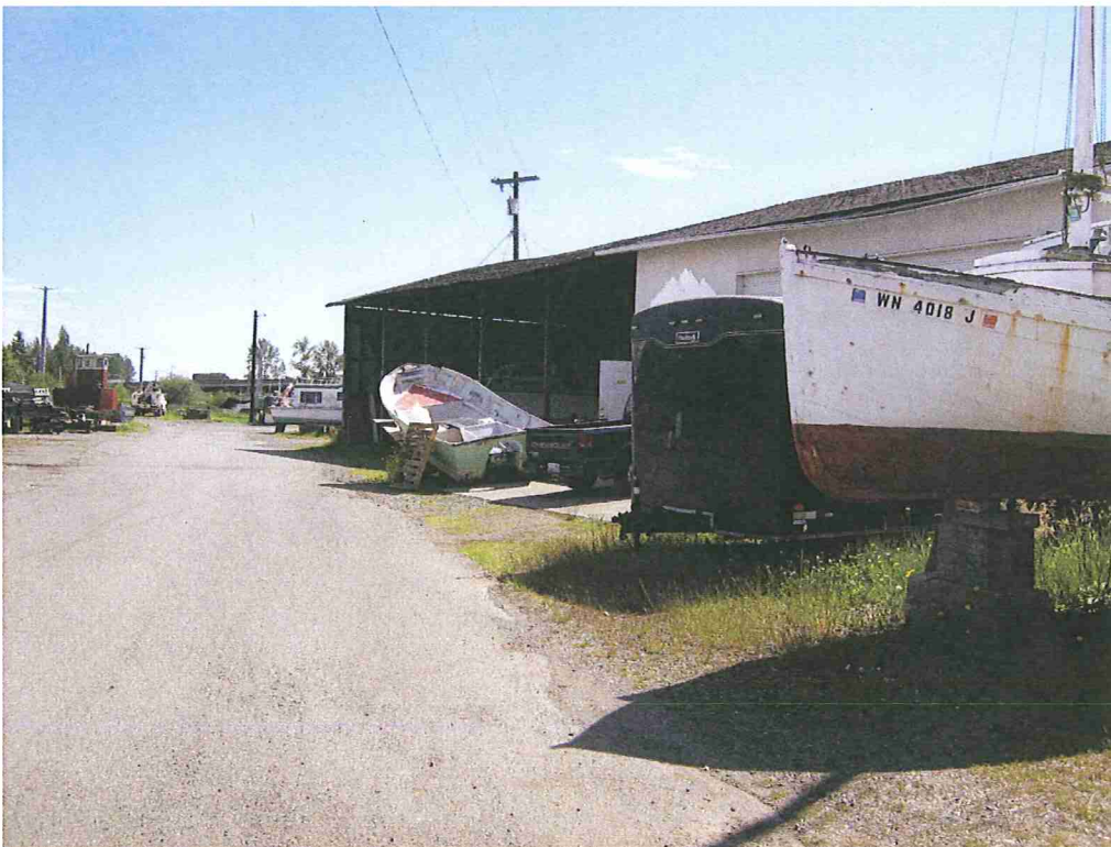
Photograph of the boat storage and workshop buildings located on the central portion of the subject property. Viewing to the southwest.
