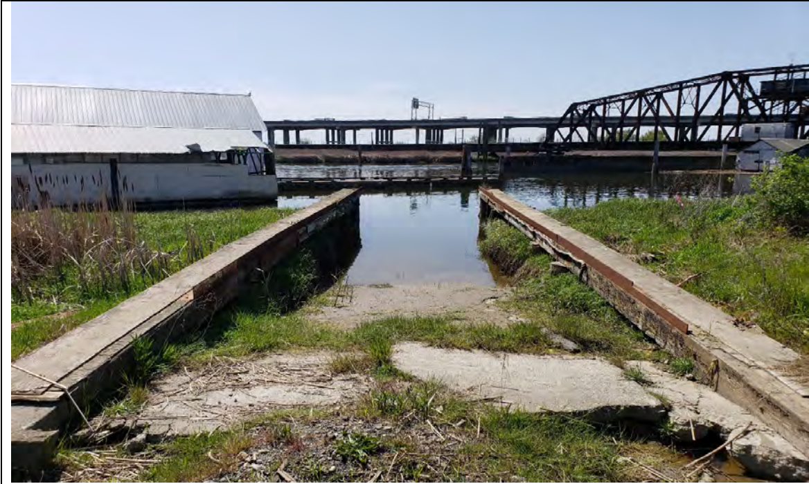
Photo 7. Old wood rail boat lift on Geddes Site in foreground extending into Ebey Slough with docks and boat houses in background. Approximate location of new non-motorized boat launch with Wetland B on either side (4/25/2018).
