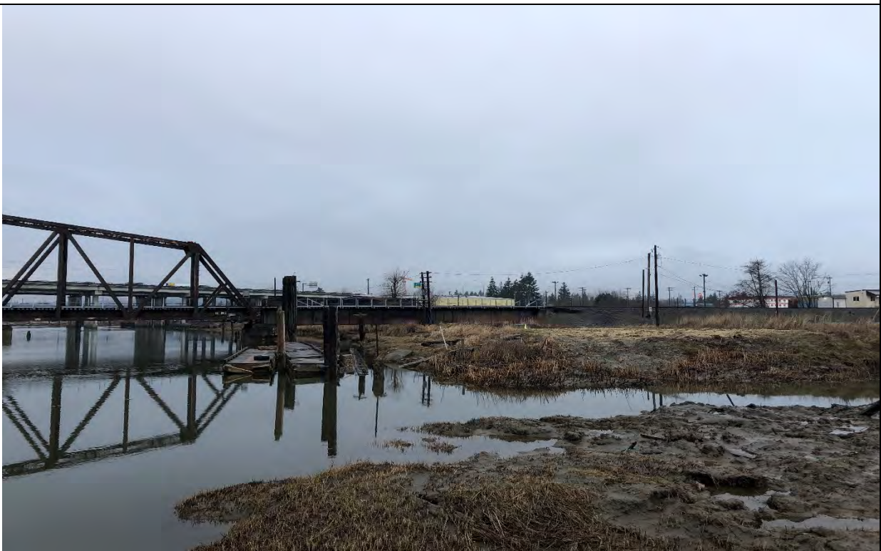
Photo 16: Remnant docks/floats/piles waterward of Geddes Site in Ebey Slough. All boat houses shown in prior pictures have been removed (3/13/2019).
