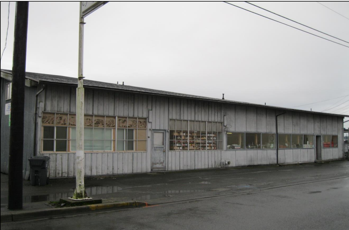
Figure 15. Overview photograph of the north side of the Geddes Marine Service building.
