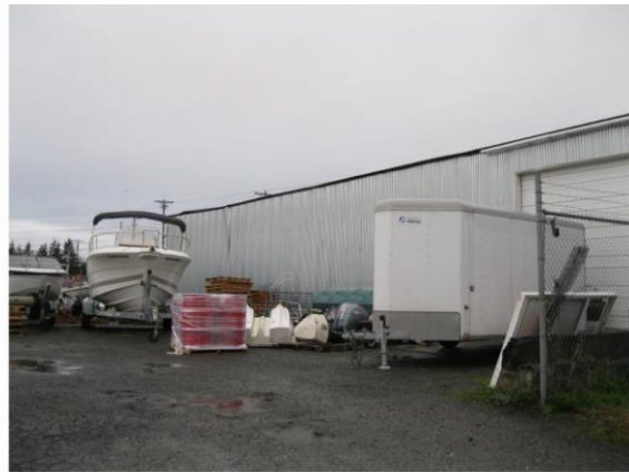
South side of building 2015
