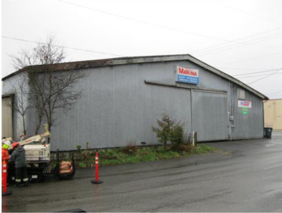
East end of building 2015
