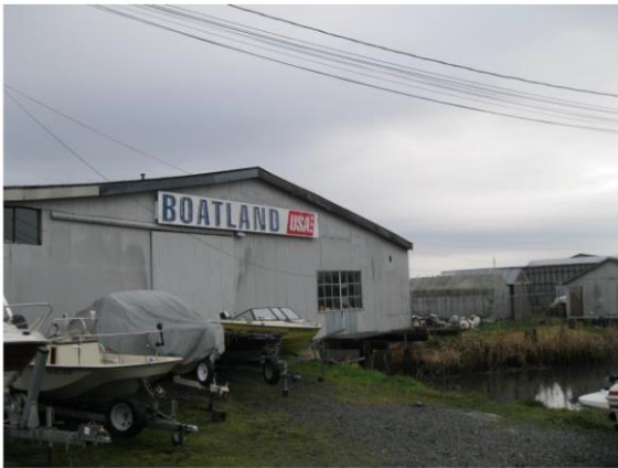
Southwest corner of building supported by pilings 2015
