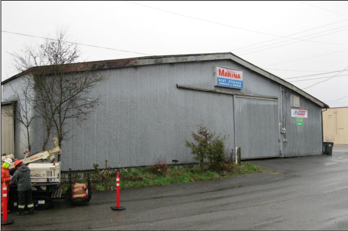
Figure 14. Overview photograph of the east end of the Geddes Marine Service building.
