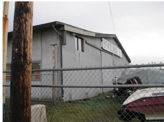
Northwest corner of building 2015
