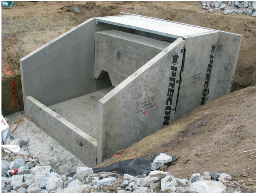
EXAMPLE CONCRETE ENERGY DISSIPATOR WITH TIDE FLEX VALVE NO SCALE
